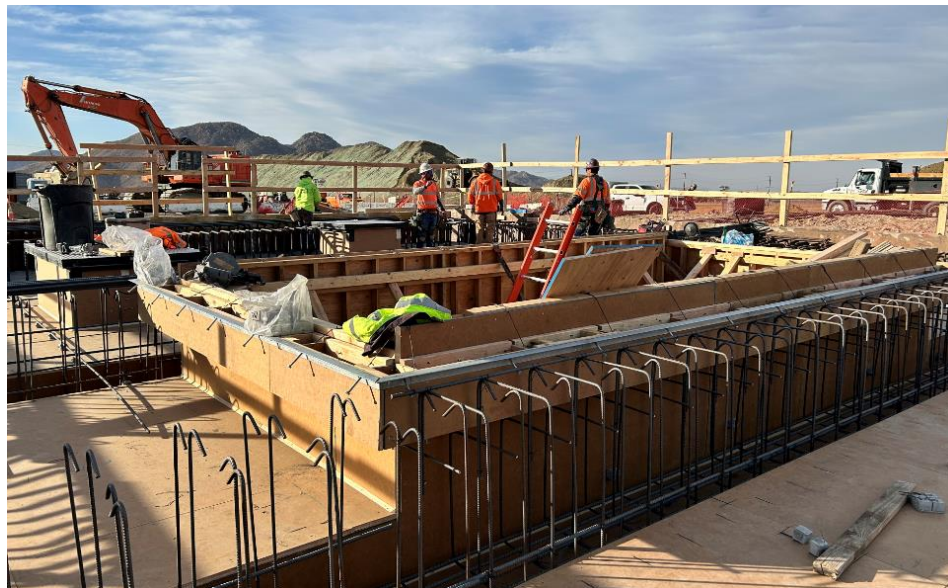
Inland Feeder-Badlands Tunnel Surge Protection—False Work Installation at Valve Vault
