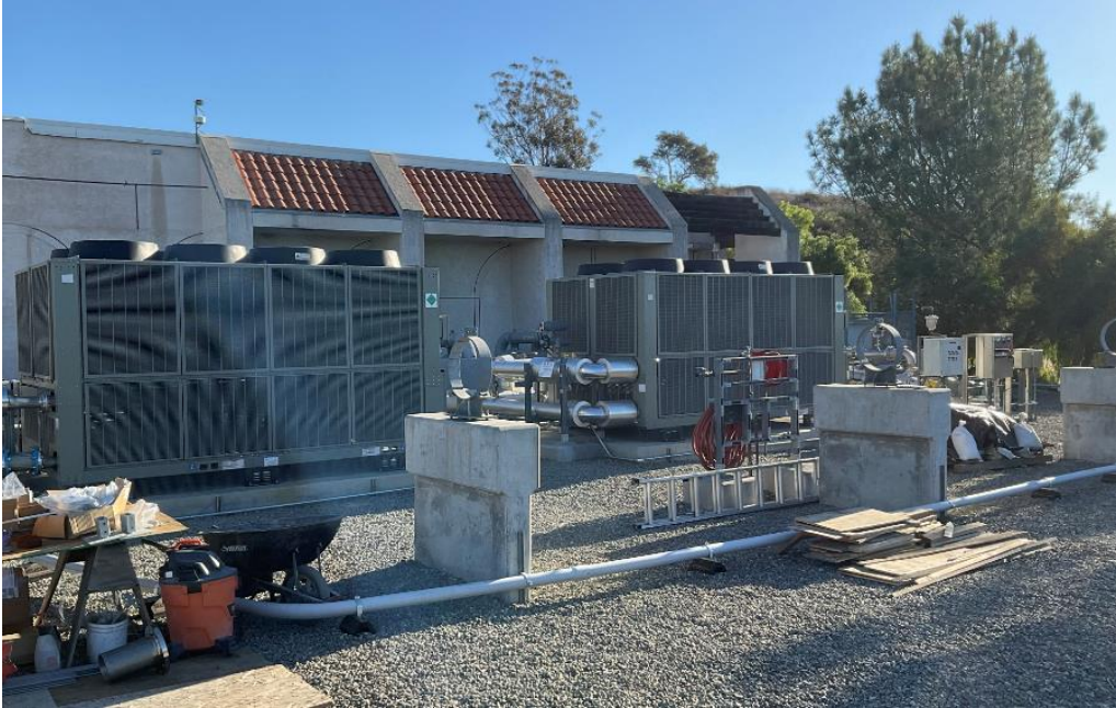
Service Connection OC-88—Replacement of two chillers
