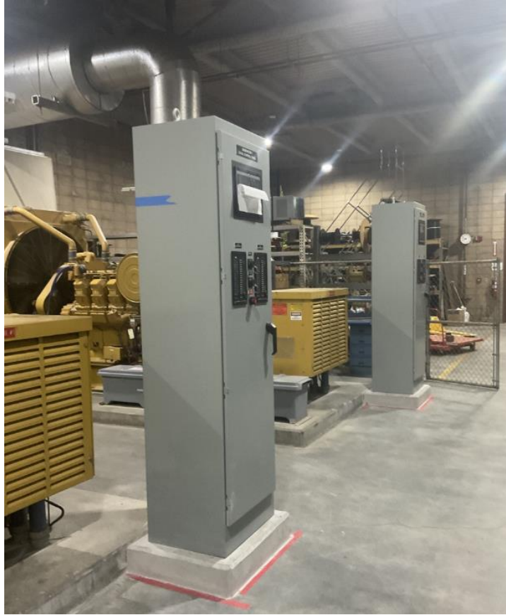
Mills Electrical Upgrades, Stage 2—New Control Panels Installed in the Engine Generator Building
