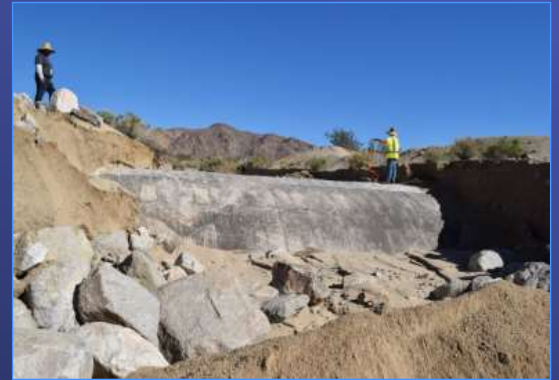
CRA Conduit Exposure from Storm (Oct. 2018)
