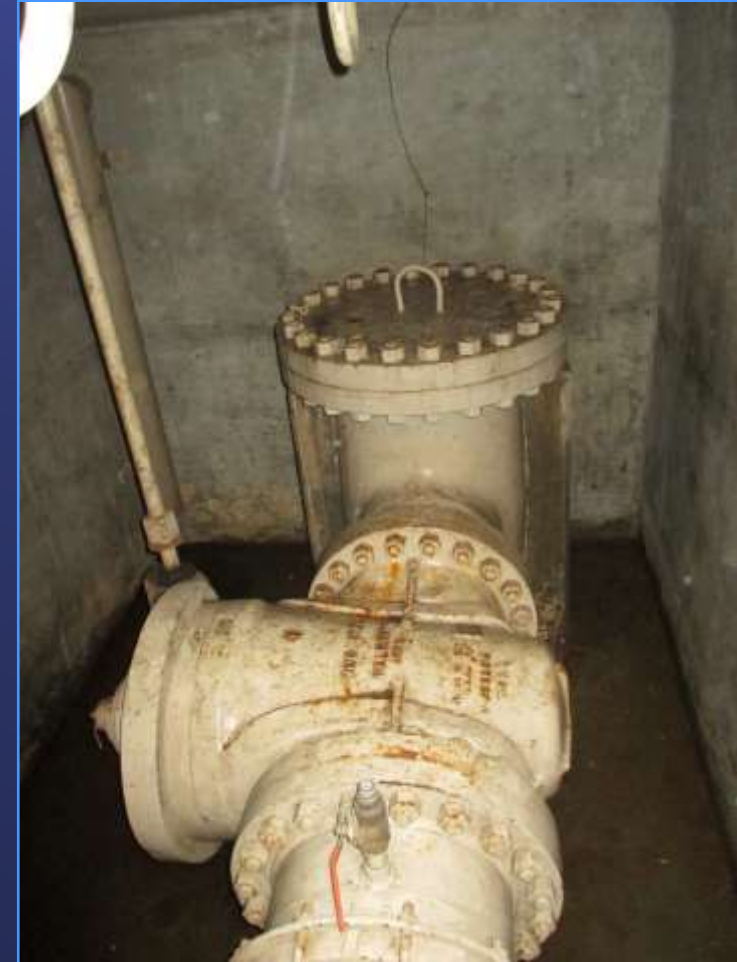
Existing deteriorated blow-off valve, typical of six
