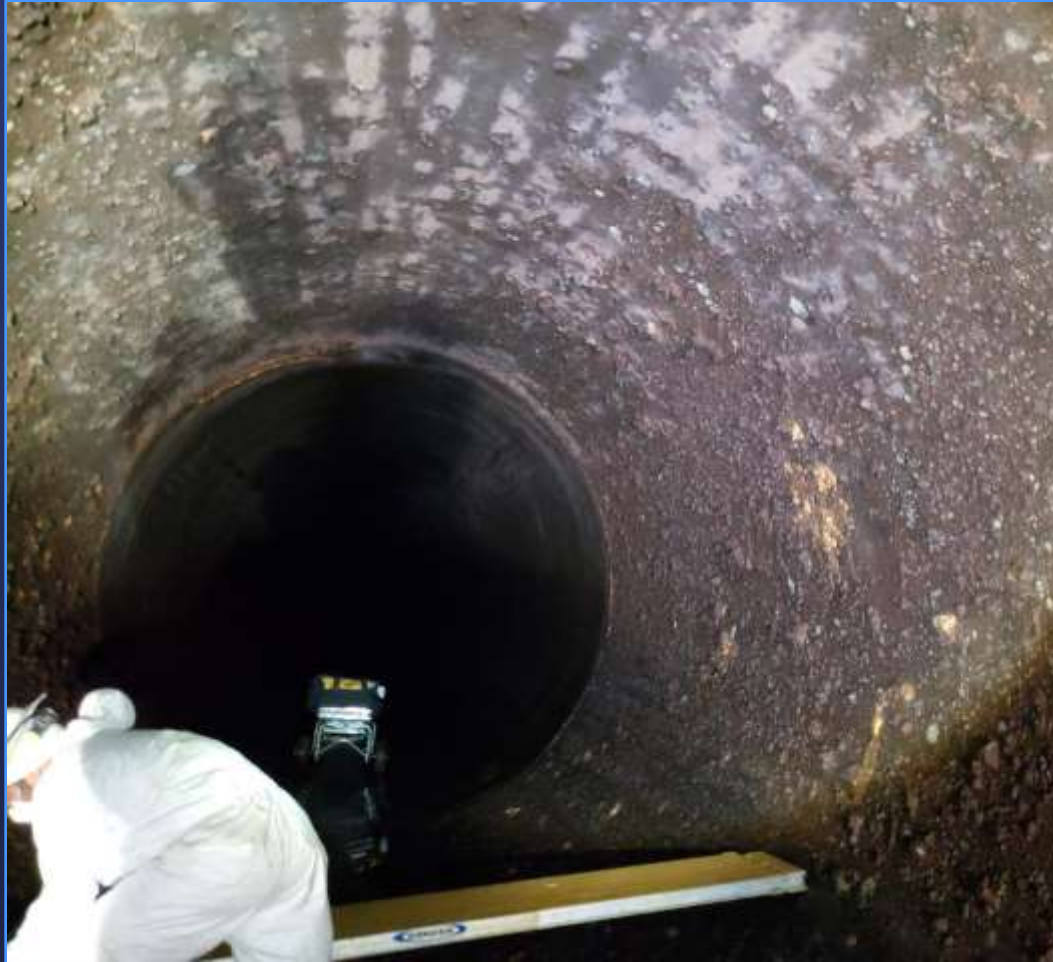
Severe corrosion and pitting in 120-inch diam. 35-ft. steel segment (Dec. 2020 inspection)
