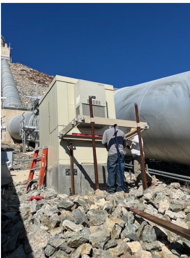
Staff installing maintenance platform (left and middle), and maintenance platform ready for painting (right)
