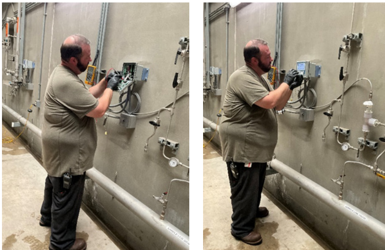
Staff working on replacing the existing ozone residual analyzer
