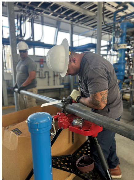
Modifying the reverse osmosis system during a week-long shutdown at the Napolitano Innovation Center demonstration plant
