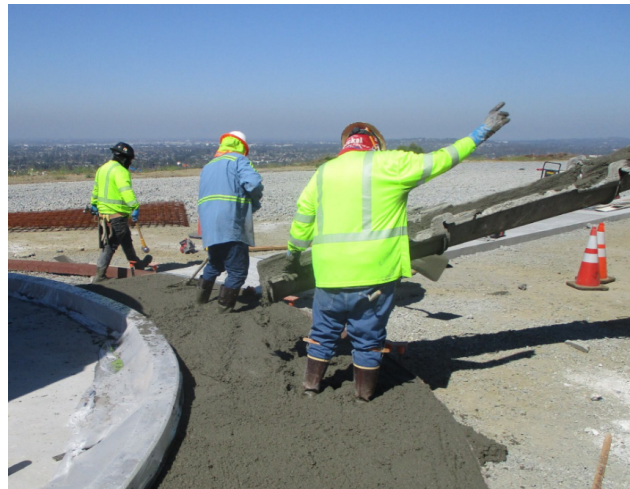
Staff installing the fire line for the heli-hydrant (left) and placing concrete sidewalk around the heli-hydrant water tank (right)
