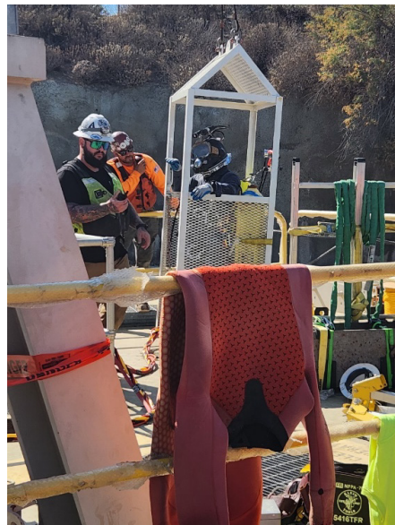
Contract diver lowered into the Lake Mathews junction shaft to inspect and clean the impacted gate
