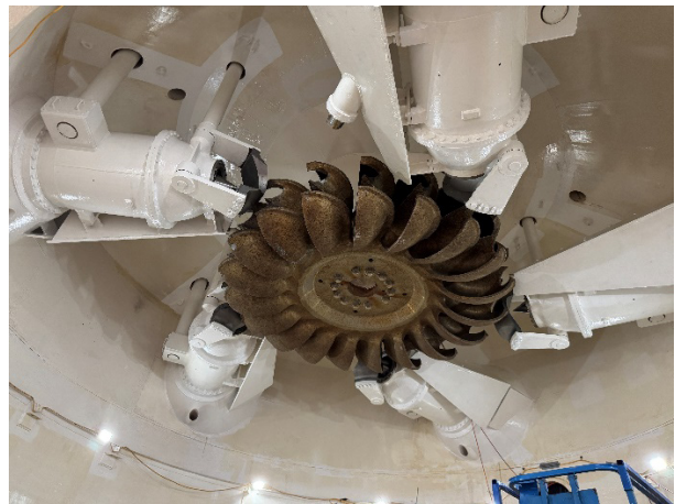
Staff installing refurbished needle valve (left) and completed needle valve installation (right) at Sepulveda HEP
