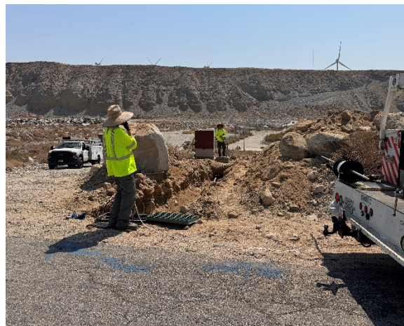
Excavating for new conduit installation (left) and installing pull rope into conduit (right) along the CRA
