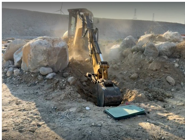
Excavating for new conduit installation (left) and installing pull rope into conduit (right) along the CRA
