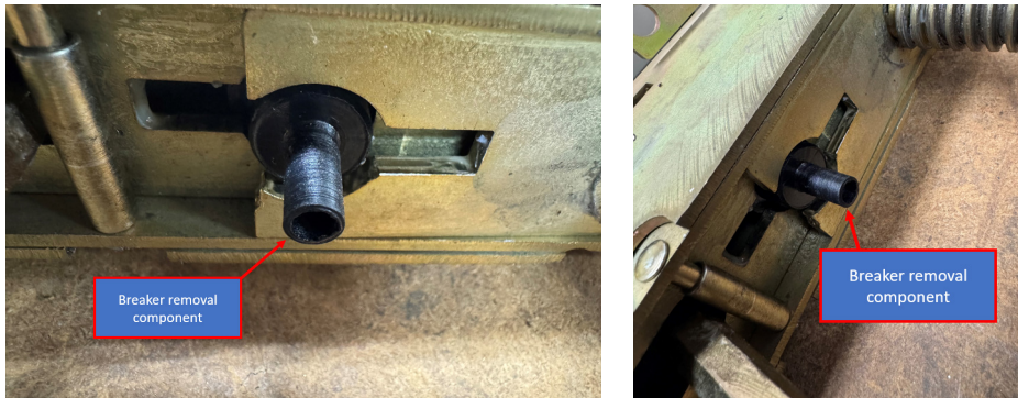
Breaker removal component for a circuit breaker at the Skinner plant
