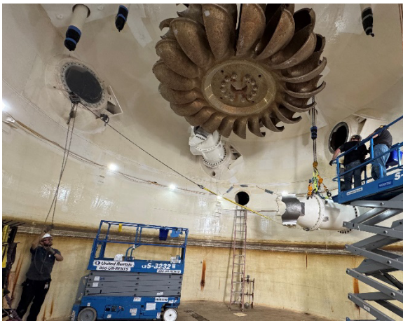
Staff installing refurbished needle valve (left) and completed needle valve installation (right) at Sepulveda HEP
