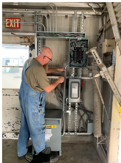
Electrician installing new equipment on a deenergized electrical panel at Hinds
