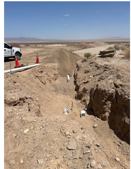
Staff laying out slope (left) and open trench (middle) for replacement sewer pipe, and new sewer pipe partially complete and backfilled (right)
