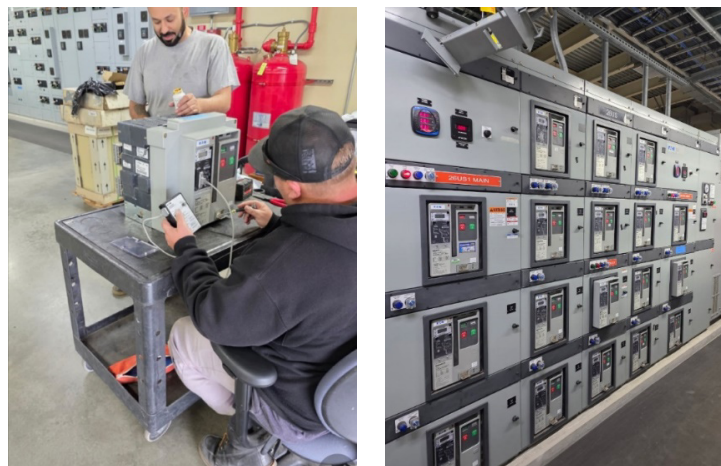
Testing circuit breakers (left) and equipment returned to service (right) at the Weymouth plant
