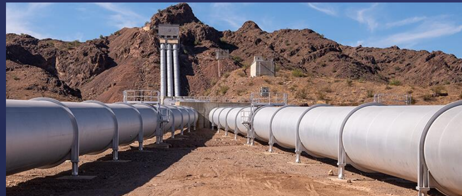
Gene Pumping Plant
