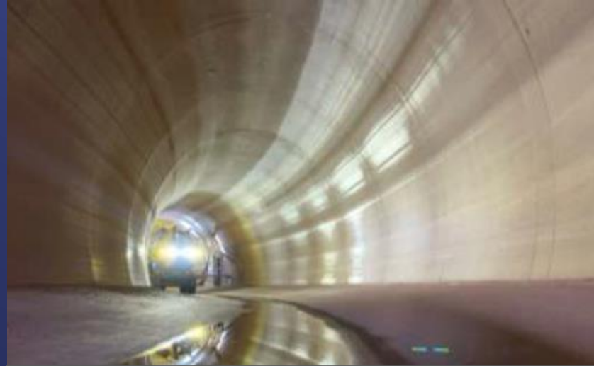
Cleaning CRA during shutdown
