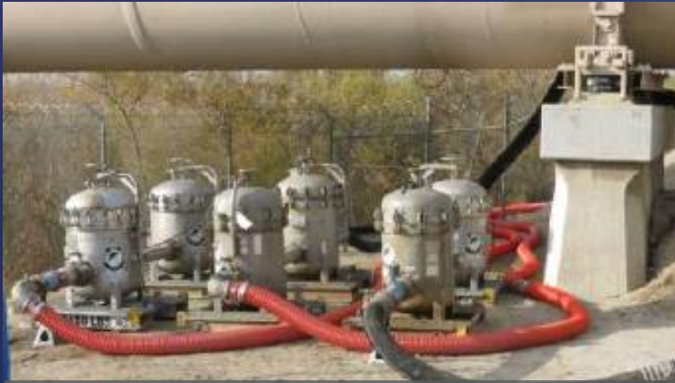
Preparation for dewatering at Upper Feeder
