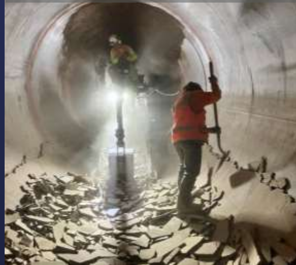
Demo of mortar lining
