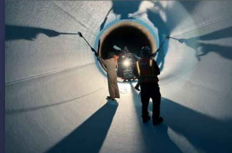
Final coating of pipe after lining repair
