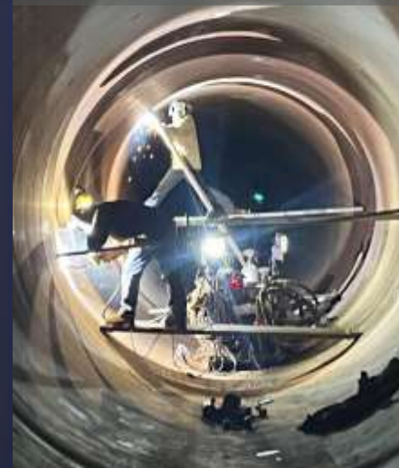
Welding steel pipe
