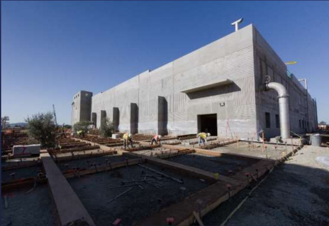
Weymouth Ozone Retrofit Project
