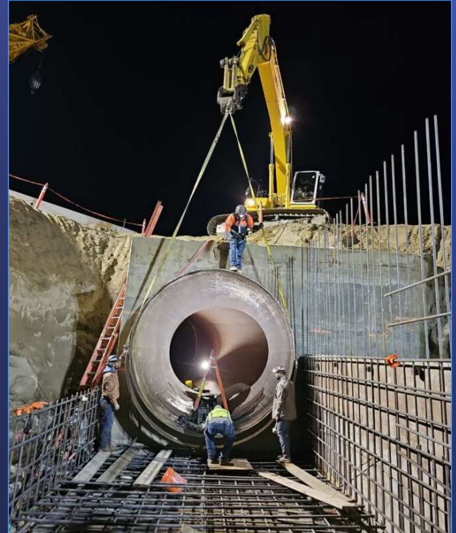
Wadsworth Bypass Shutdown work
