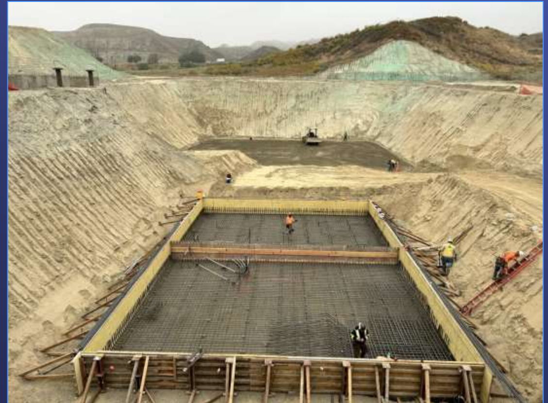
Installation of formwork and rebar at project site
