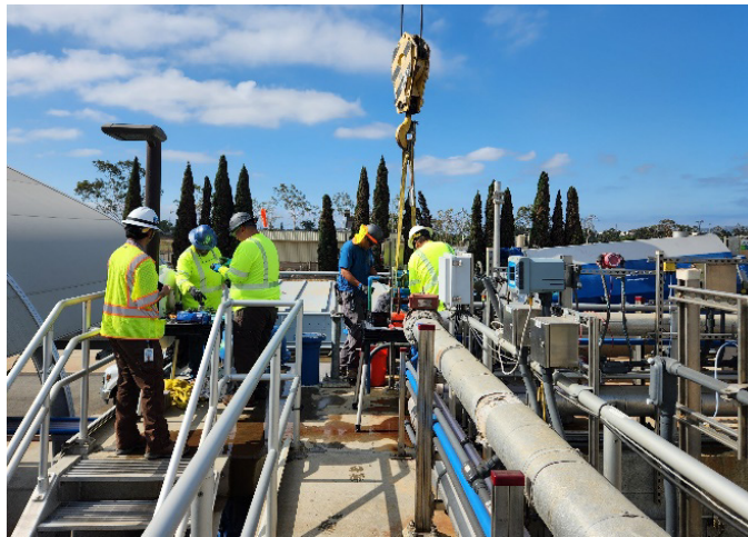
Staff replacing the influent valve at the demonstration facility.
