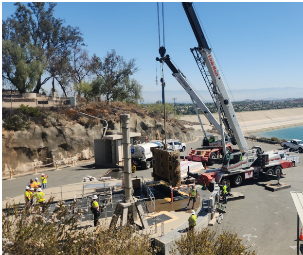
Junction Shaft gate as it clears the top of the shaft (left), and being laid down on cribbing using two cranes (right) at Lake Mathews.
