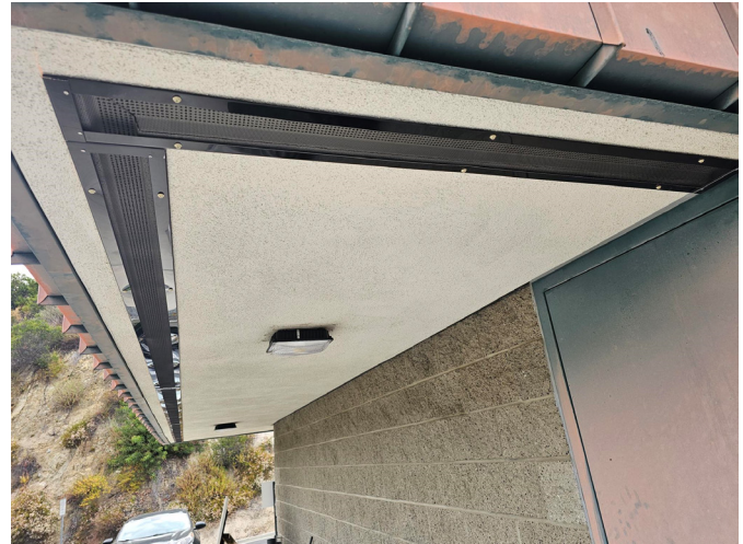
Staff installing ember-resistance screens (left) and installed vent screens (right).
