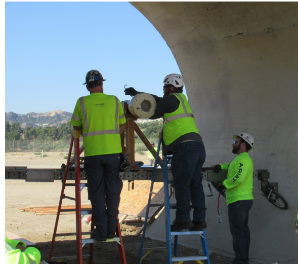
Staff exposing layers of steel wires on the pipe exterior (left) and inspection equipment being installed for the calibration test (right).
