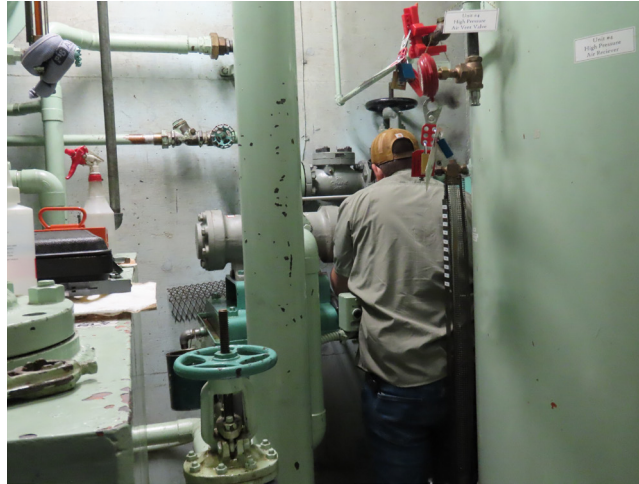
Staff replacing Hinds Unit 4 discharge valve high-pressure pump.
