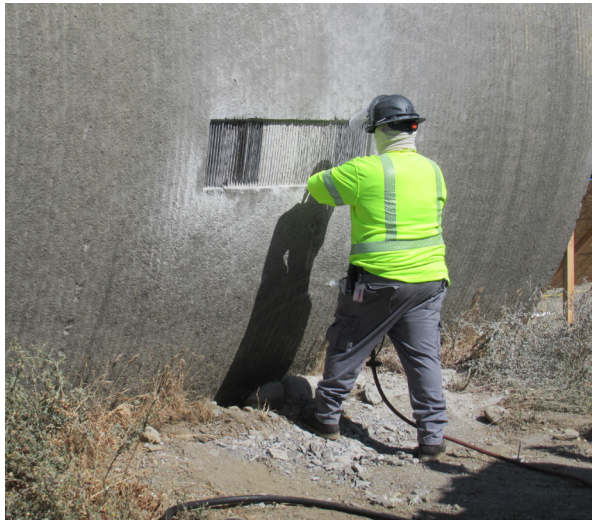
Staff exposing layers of steel wires on the pipe exterior (left) and inspection equipment being installed for the calibration test (right).
