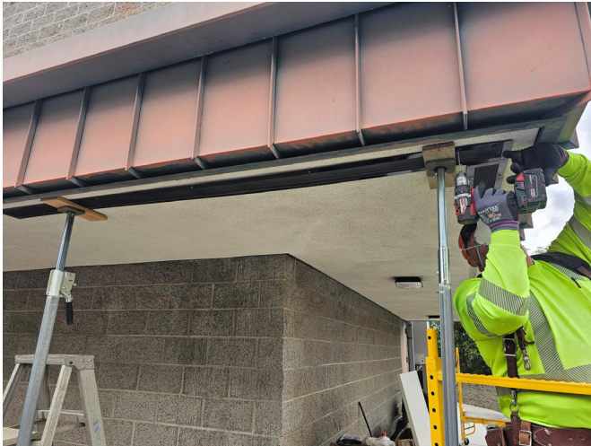
Staff installing ember-resistance screens (left) and installed vent screens (right).
