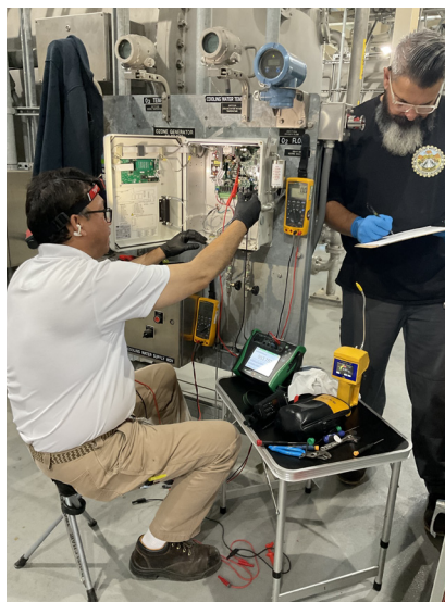
Staff gathering data prior to making ozone analyzer adjustments at Weymouth plant.
