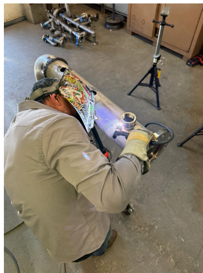
Staff fabricating new stainless-steel piping at Eagle pump plant.
