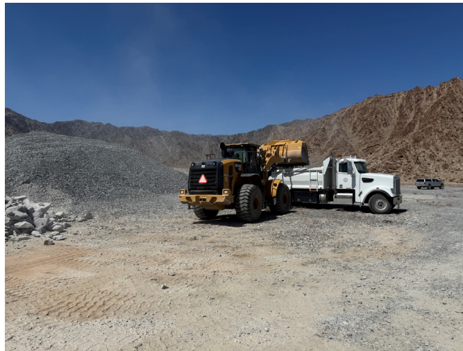
Staff hauling aggregate for CRA road repairs.
