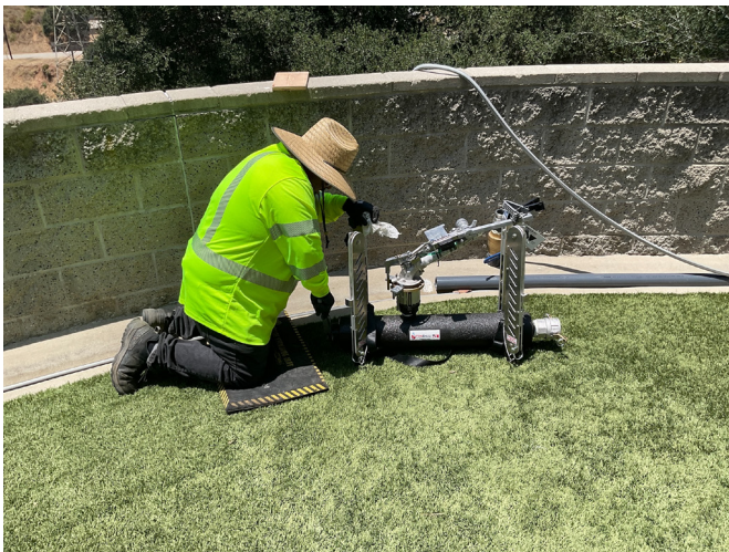
Staff installing high-intensity sprinklers (left) and supply pipe installation (right).
