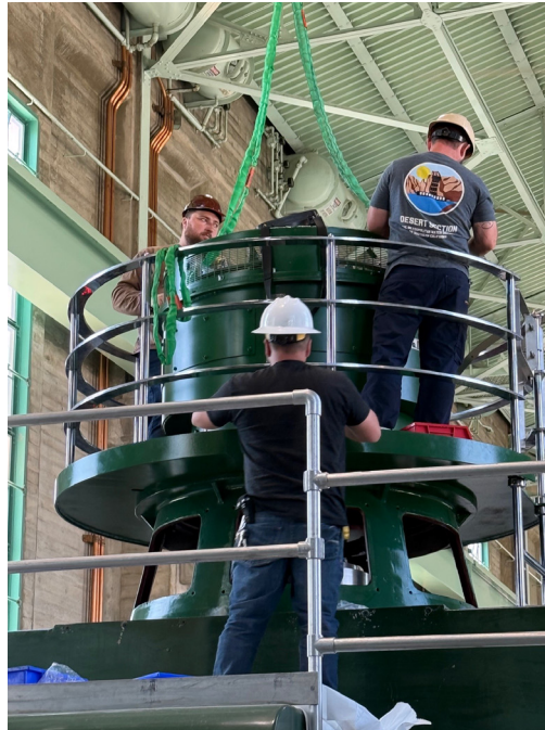
Staff installing new brushless excitation components on Gene Unit 1.
