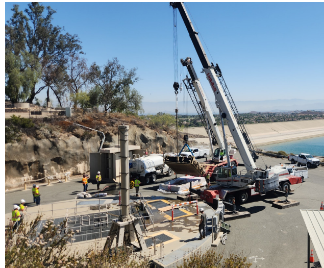
Junction Shaft gate as it clears the top of the shaft (left), and being laid down on cribbing using two cranes (right) at Lake Mathews.
