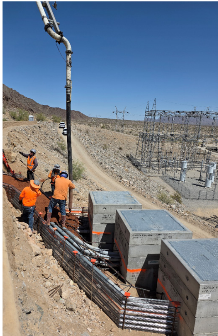
CRA Domestic Water Treatment System at Hinds Pumping Plant — Placing Concrete for Ductbank
