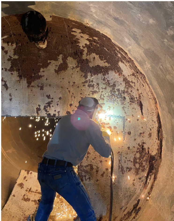
Perris Valley Pipeline Tunnels — Welder Cutting Bulkhead
