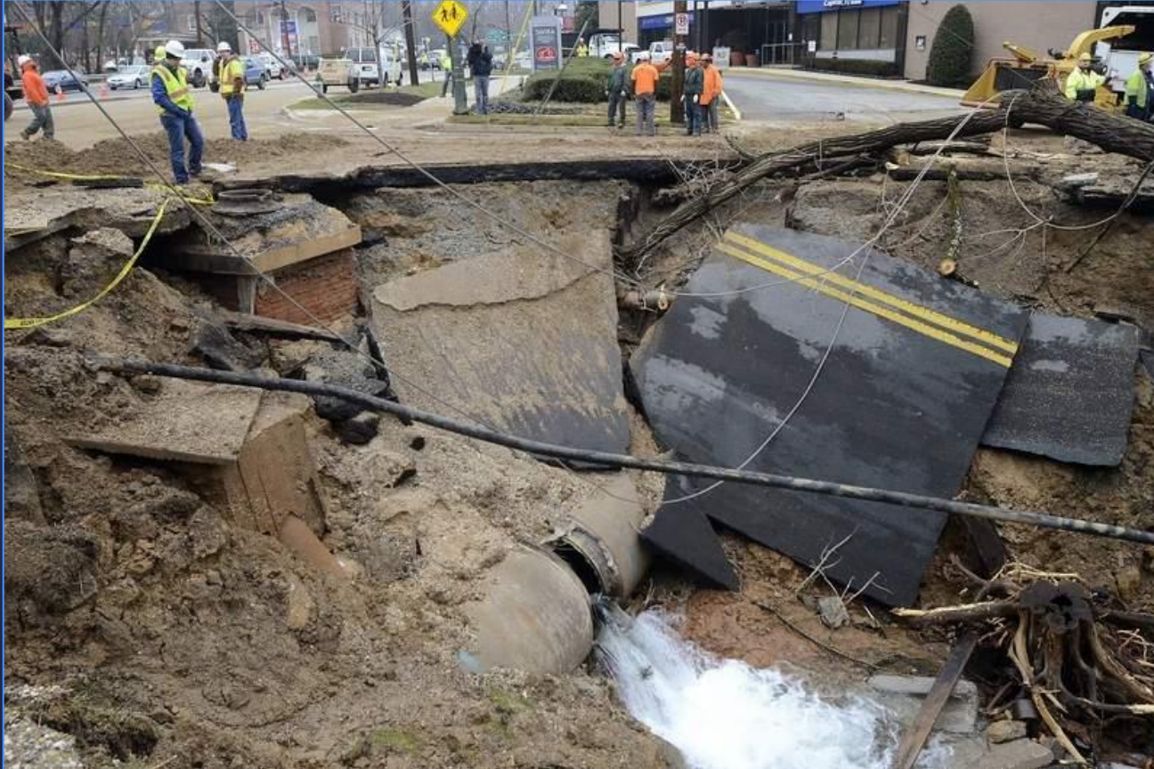
Washington Suburban Sanitary Commission 60" PCCP Failure 2013
