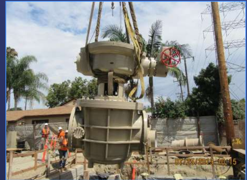
42-inch diameter sectionalizing valve for Second Lower Feeder
