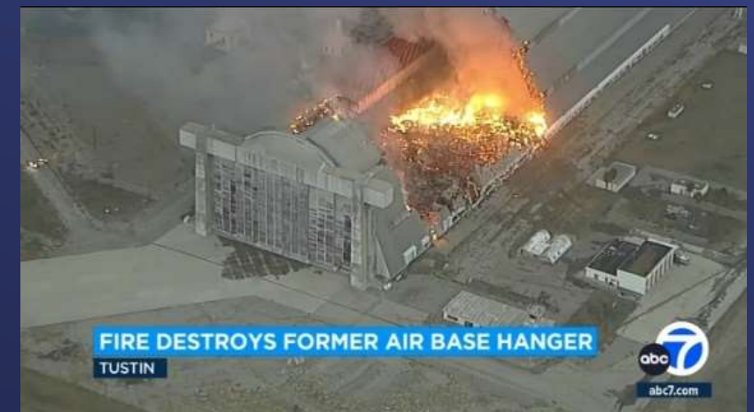
OC Hangar Fire November 2023
