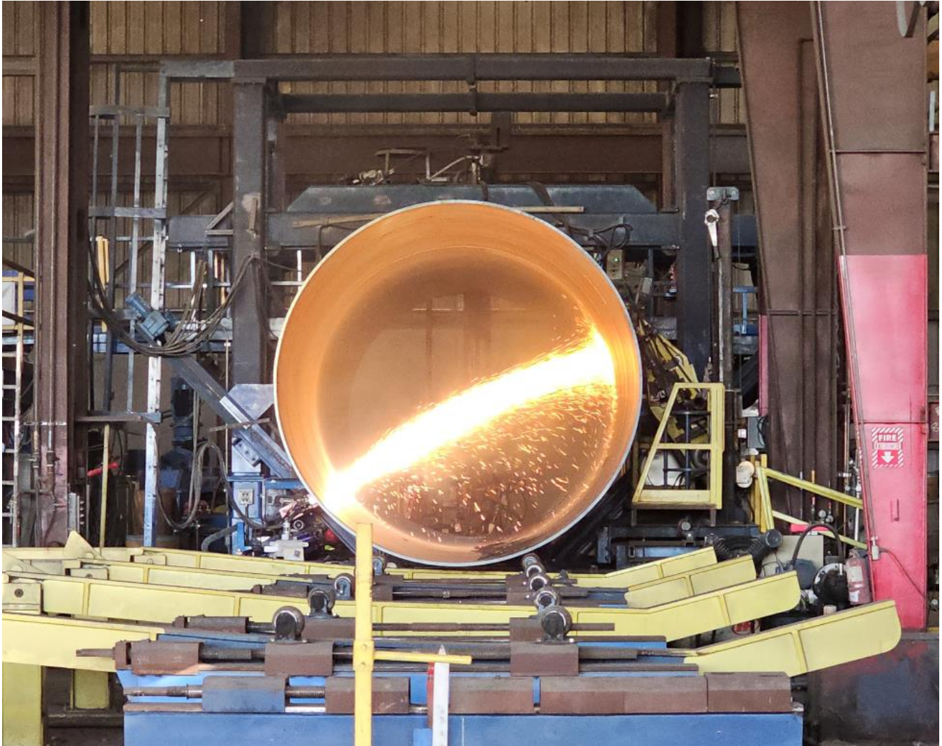
Lakeview Pipeline Relining-Procurement—Plasma Torch Cutting of 117-inch Diameter Pipe
