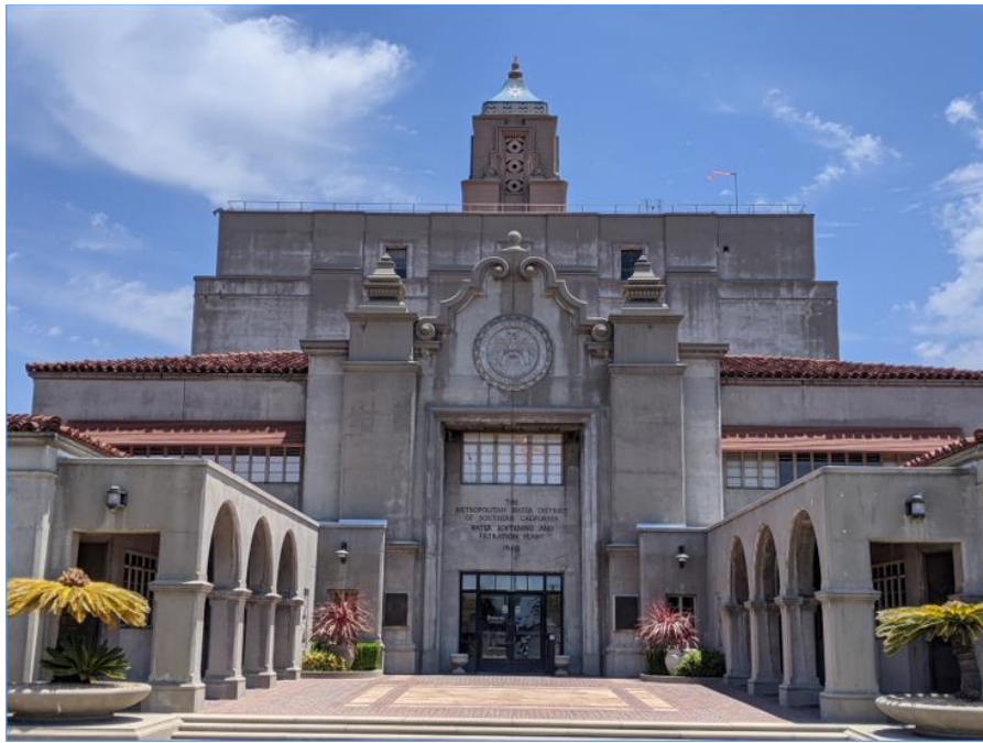
Weymouth Water Treatment Plant – Administration Building
