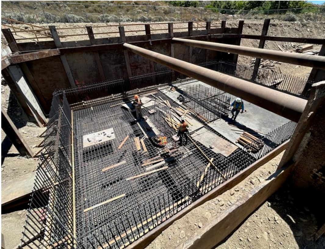
Inland Feeder-Rialto Intertie—Placing Reinforcing Steel for the Valve Vault Foundation
