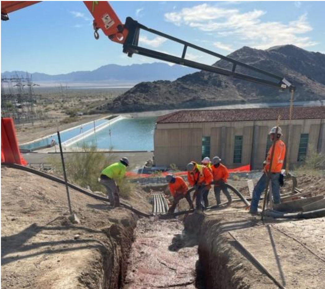
Domestic Water System Upgrades—Ductbank to Domestic Tank at Eagle Mountain
