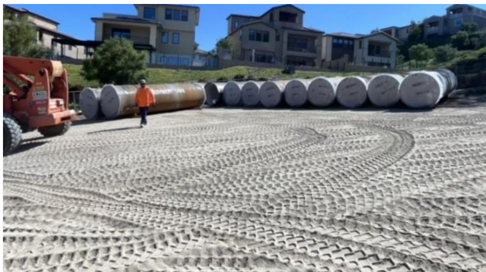
Allen-McColloch Pipeline Urgent PCCP Rehabilitation—Pipe Laydown Area at Pipe Access Site
