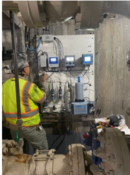
Staff working on a water quality panel at the Beverly Hills Pressure Control Structure
