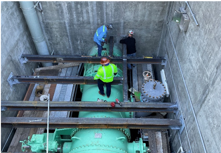
Staff mounting I-Beams to structure walls (left) and 100-ton crane hoisting I-Beams (right) at OC-88 valve structure along the AMP
