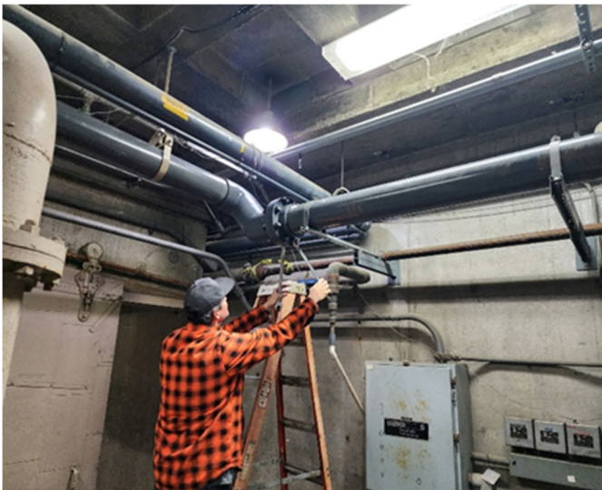
Staff assembling supply piping (left) and checking for leaks (right) at the Weymouth plant
