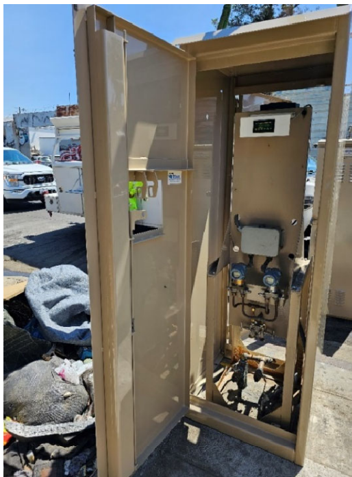
Automated Meter Reading (AMR) billing meter cabinet
