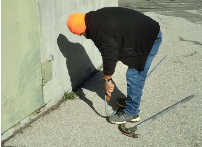
Staff installing electrical conduit at Magazine Canyon Junction Shaft
