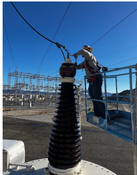
Staff testing the 230kV transformers at Eagle Mountain pumping plant
