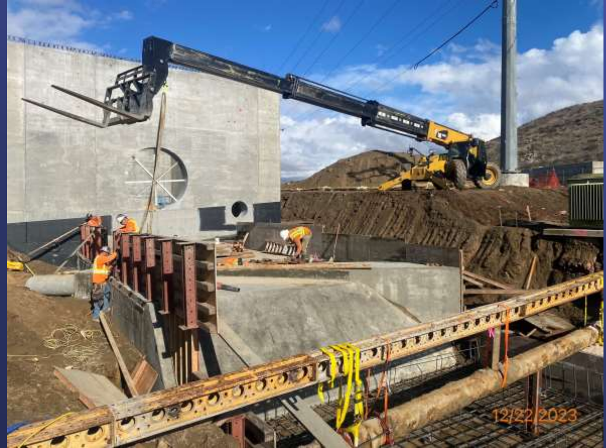
New Vault Structure
