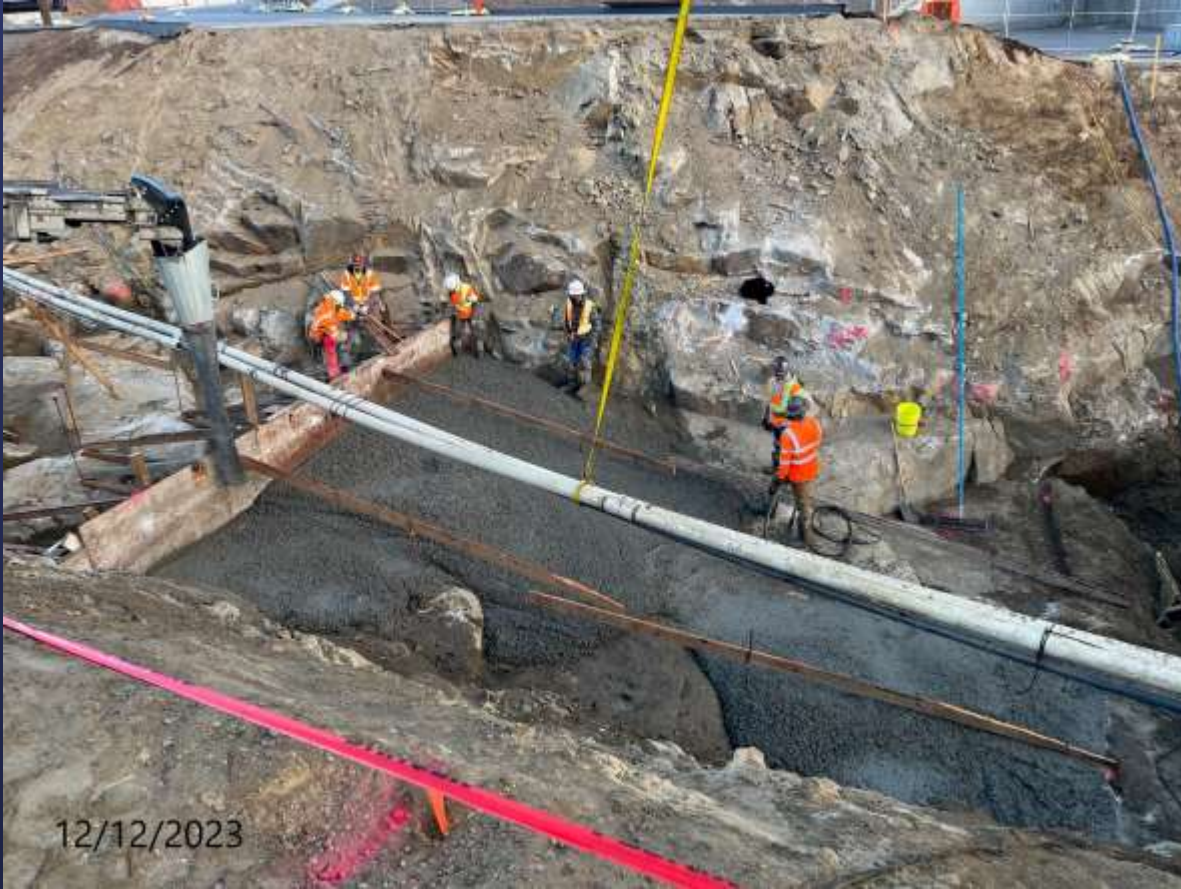
Pouring of Mass Concrete at 96" Pipe Tie-in
