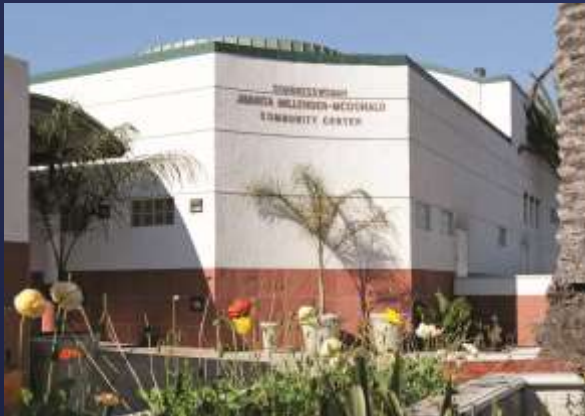
Carson Events Center
