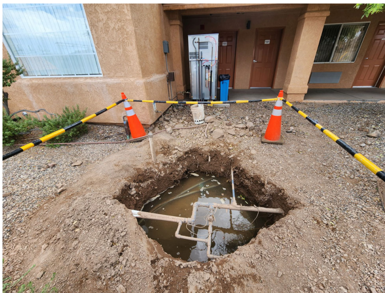
Plumbing staff repaired a leak in the fire water system.
