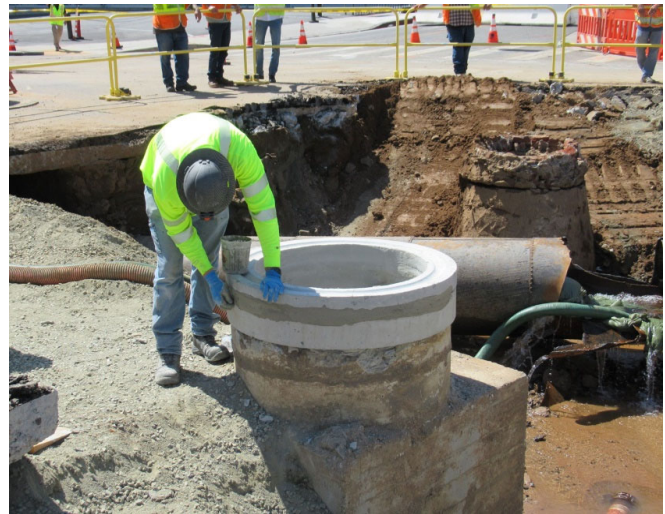
Damaged blowoff structure (left) and staff repairing damaged blowoff structure (right) on the Santa Monica Feeder.
