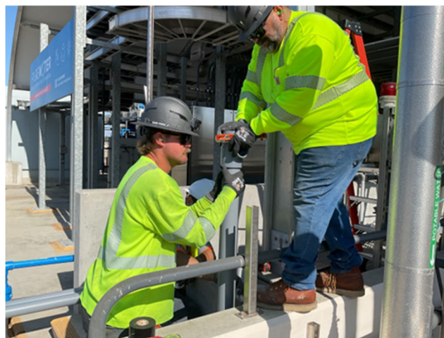
Staff installing supports and piping for the above-ground potable water system at the Napolitano Innovation Center.
