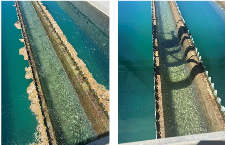
Module 3 Launder and Basin Cleaning
