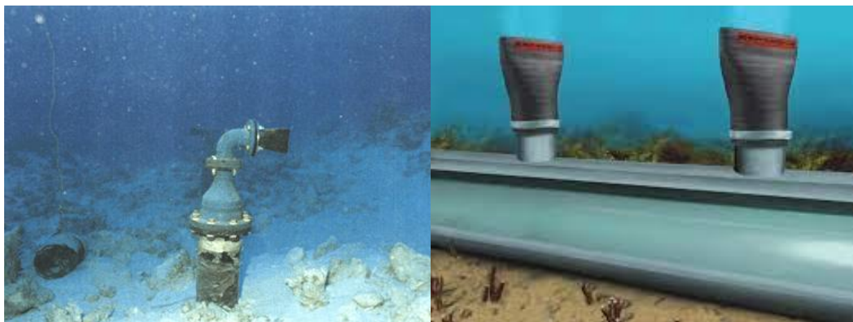
Figure 3.23 Tideflex Duckbill Diffusers in Ocean Outfall (Courtesy of Red Valve)
