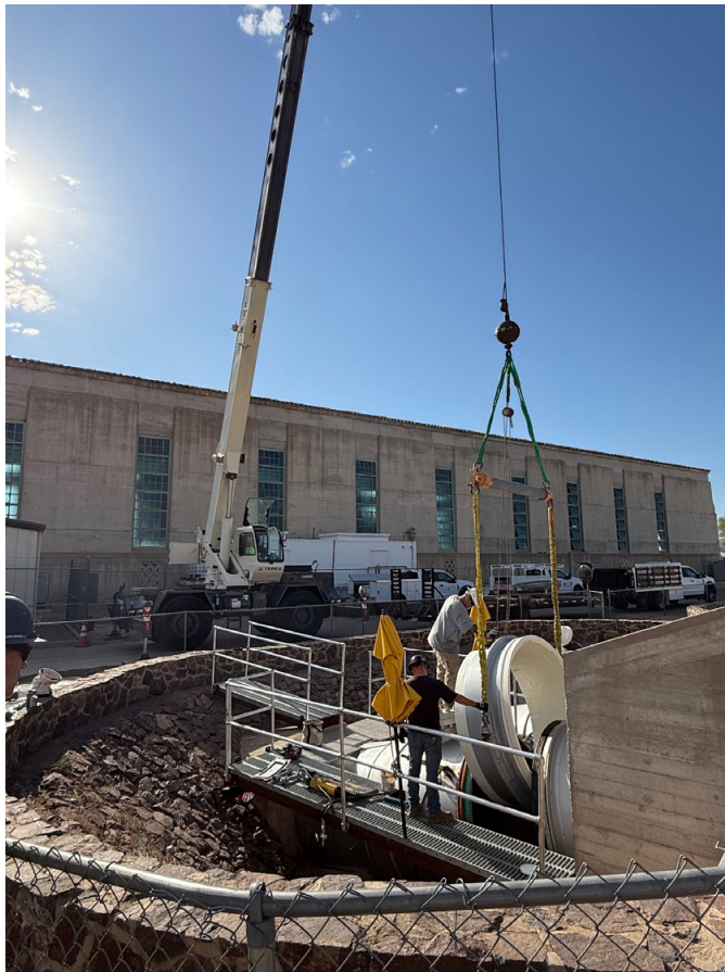
Staff removing Gene Unit 1's pant leg isolator.
