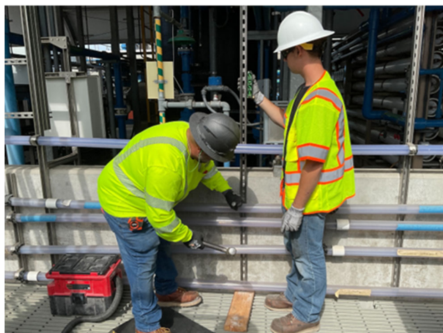
Staff installing supports and piping for the above-ground potable water system at the Napolitano Innovation Center.
