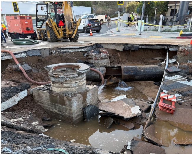
Damaged blowoff structure (left) and staff repairing damaged blowoff structure (right) on the Santa Monica Feeder.
