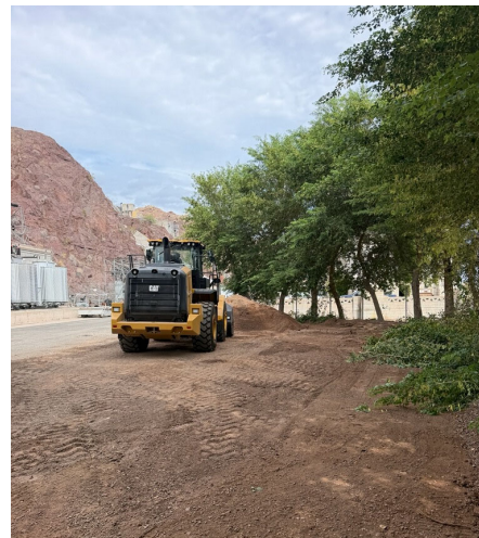
Staff removing trees (left) and grading for concrete barrier installation (right).
