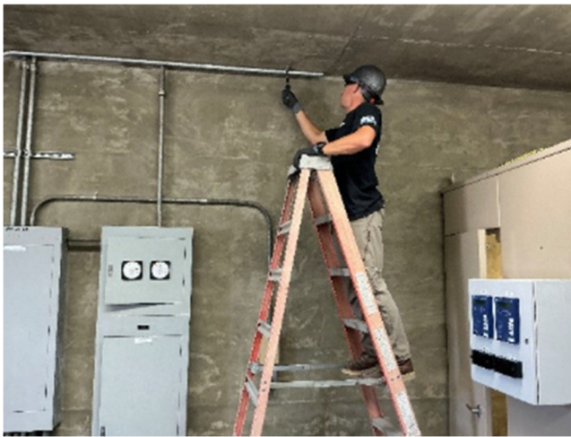
Staff installing conduit (left) and enclosure (right) for improved communication systems at Rio Hondo HEP.
