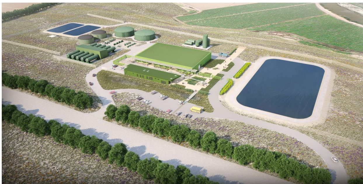
Figure 6.3 Monterey Seawater Desalination Plant
