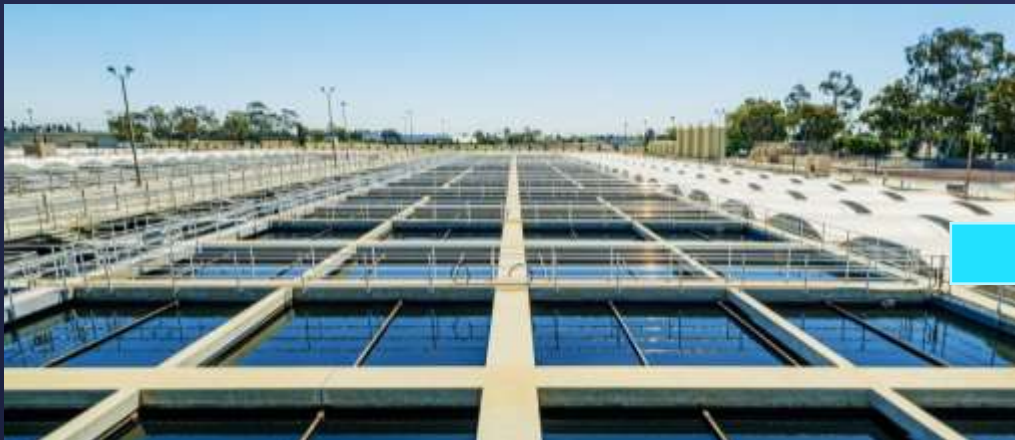
A.K. Warren Water Resource Facility
