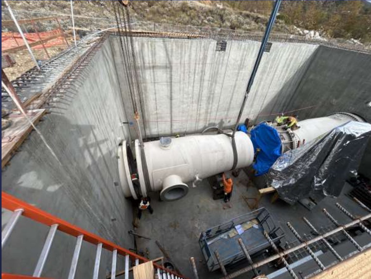
Pipe Reducer Installation
