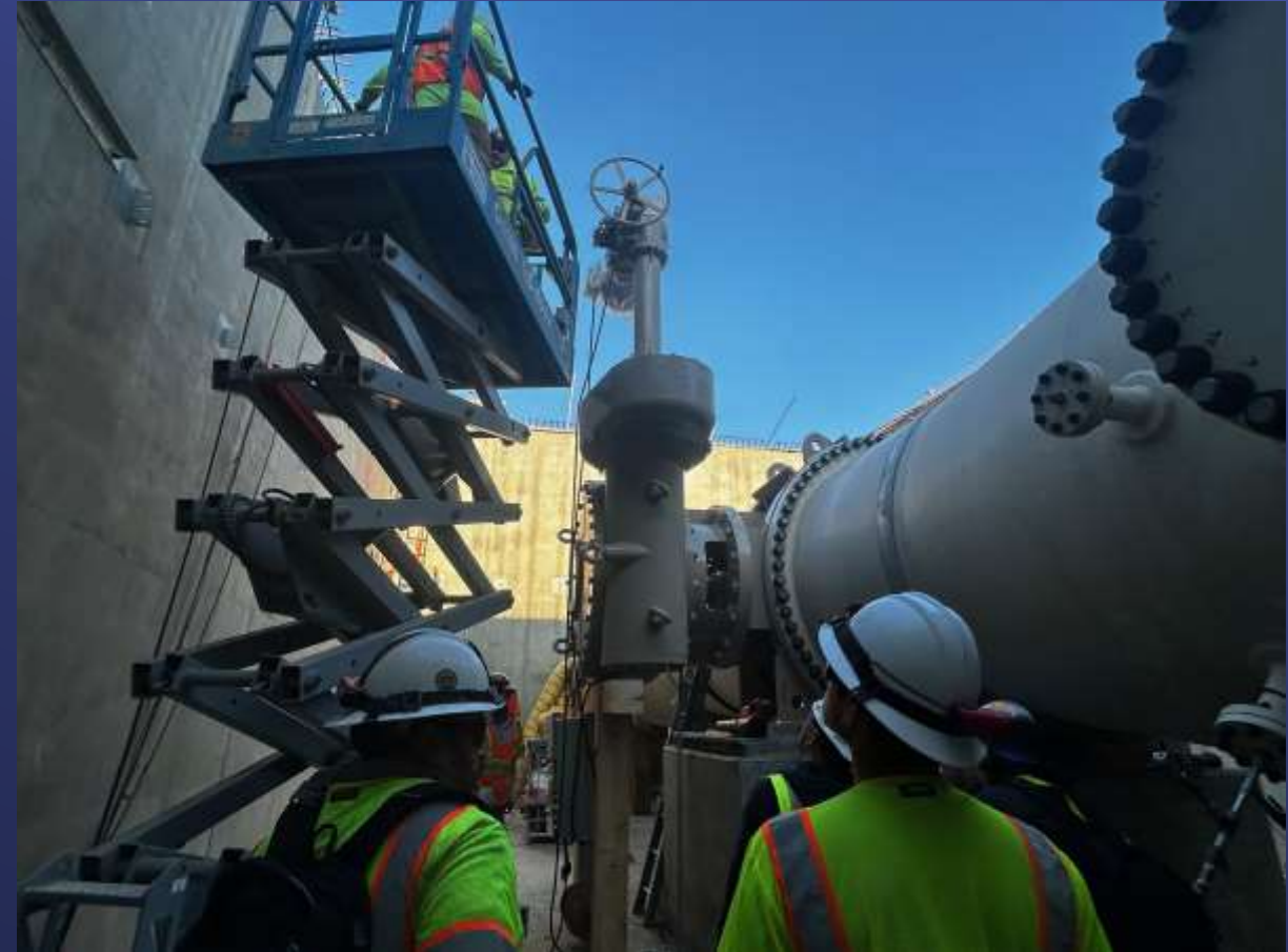
84-Inch Diameter Valve Fit Up
