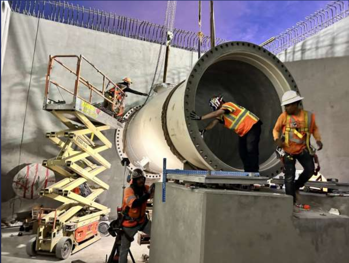
Valve Vault Pipe Installation
