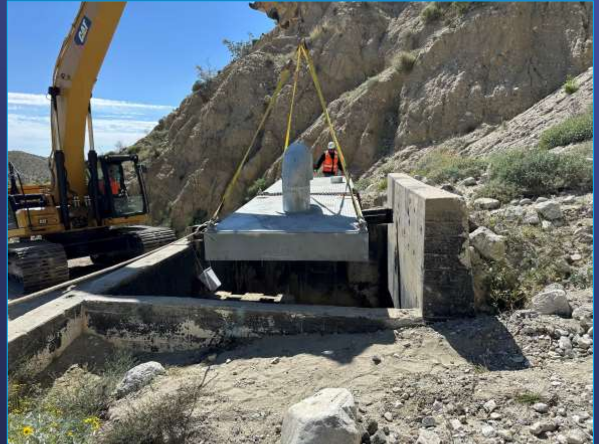
CRA Conduit Protection – Transition Cover Installation
