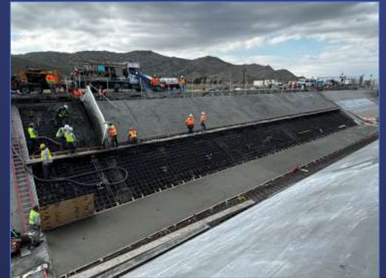
San Diego Canal Rehabilitation Stage 3 – Replacement of Concrete Liner
