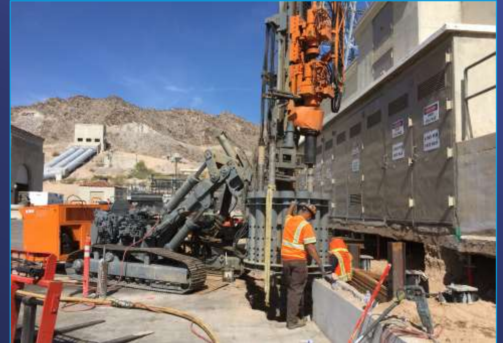
CRA 6.9kV Switch House Seismic Upgrades – Drilling for Micropiles
