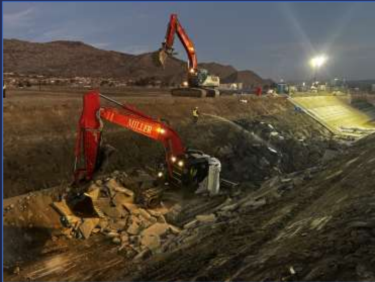
San Diego Canal Rehabilitation Stage 3 – Replacement of Concrete Liner
