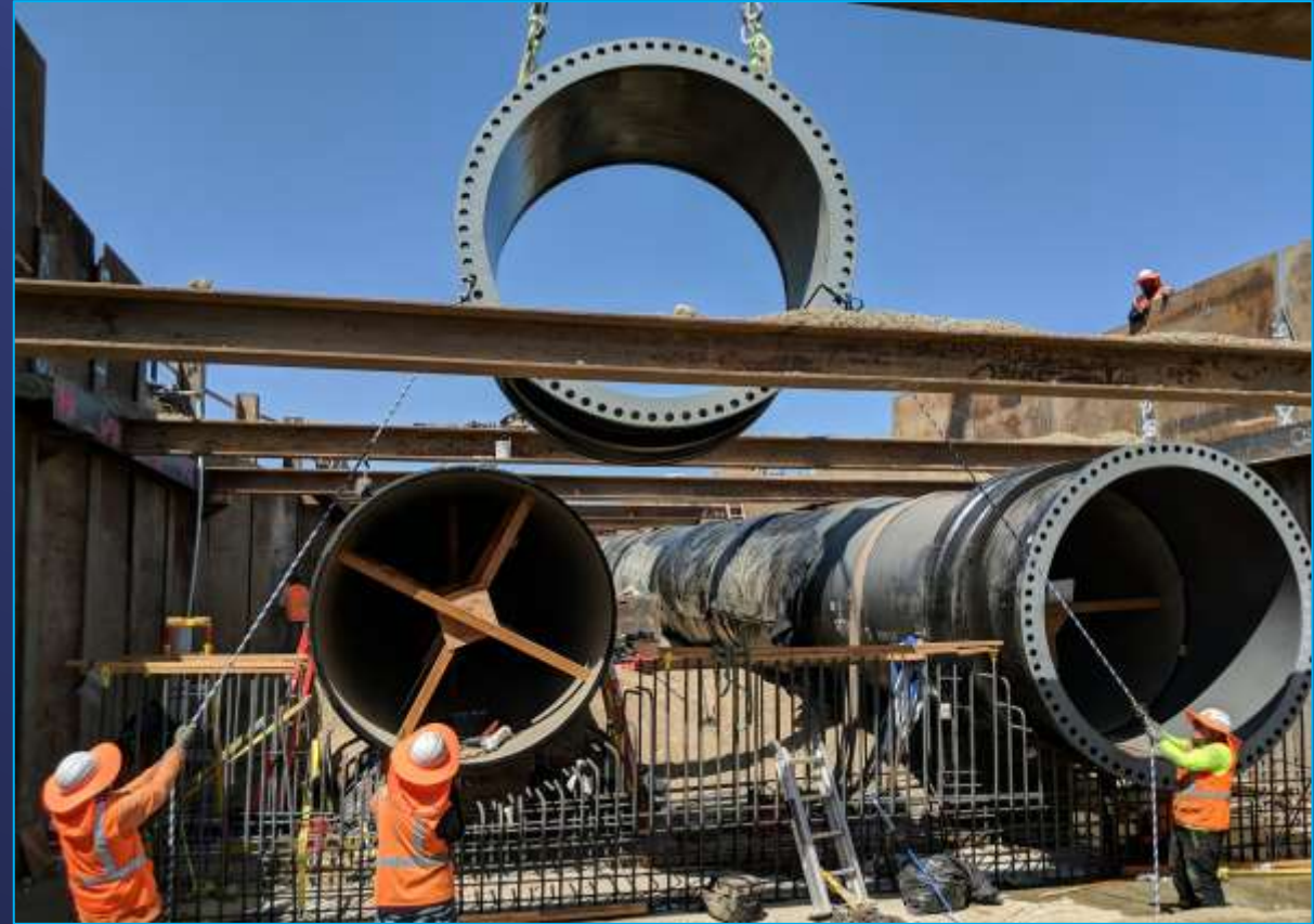
Casa Loma Siphon – Installing Earthquake Resistant Ductile Iron Pipe (ERDIP)
