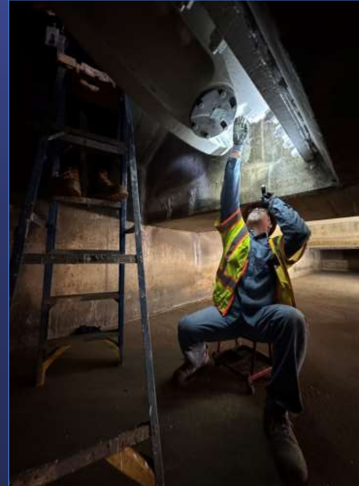
Weymouth WTP Basins 5-8 – Inspection of Valve Coating
