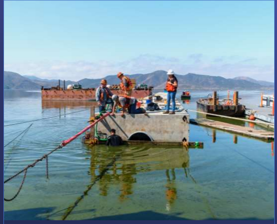
DVL Floating Wave Attenuator – Concrete Module Repair
