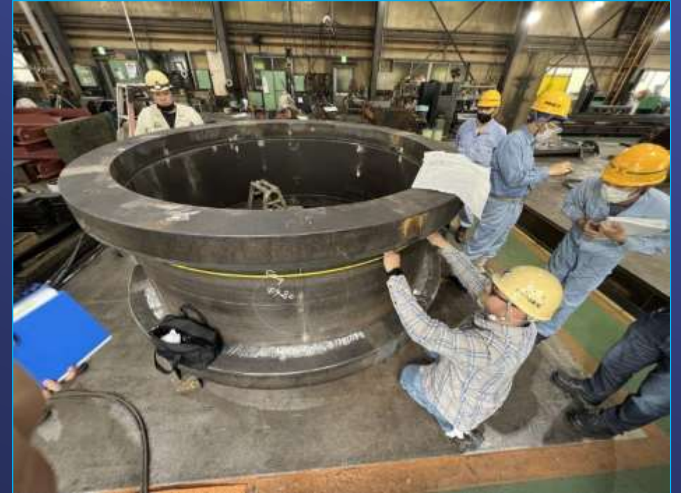
Off-site Fabrication Inspection – 84-inch Valve for Wadsworth Pumping Plant
