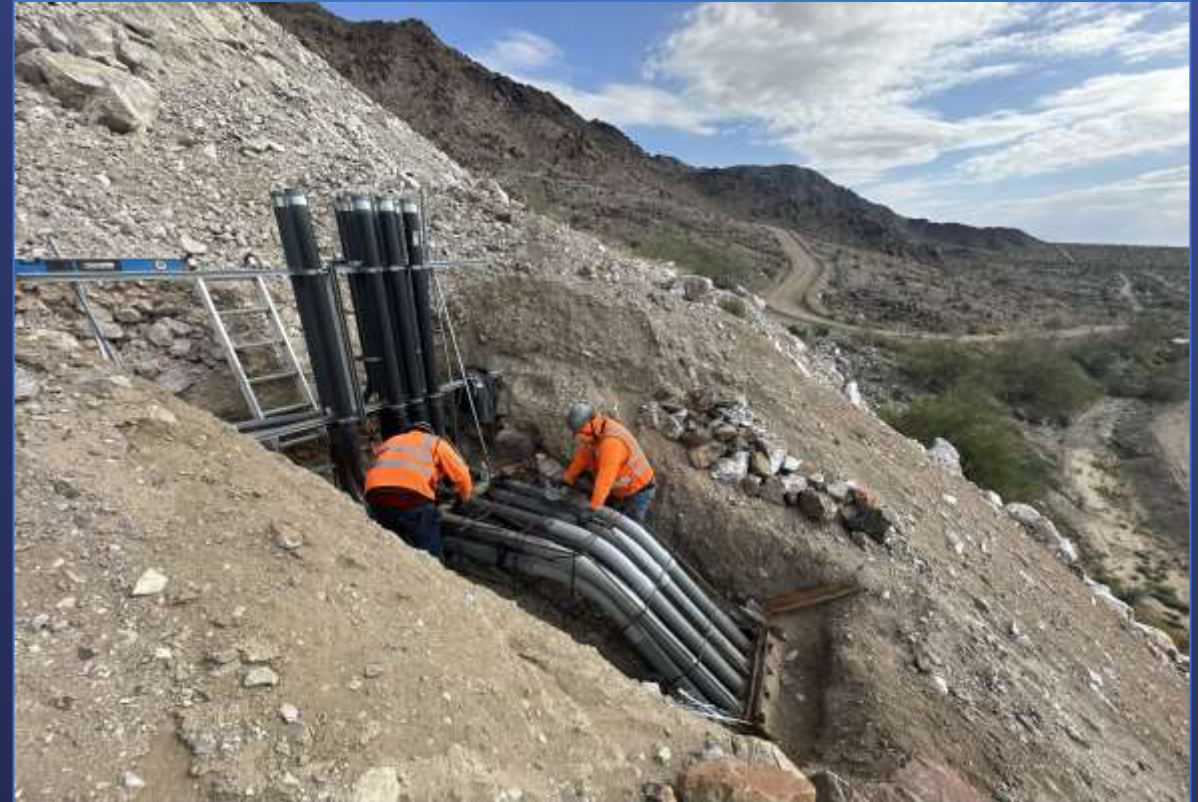
CRA Domestic Water Treatment System Replacement – Electrical Ductbank
