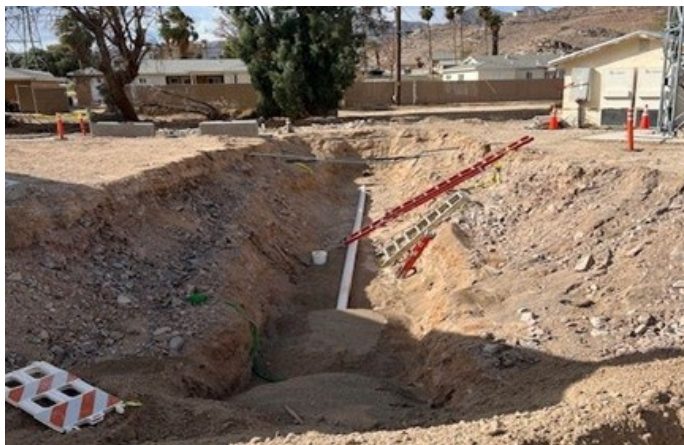
Iron Mountain sewer line replacement
