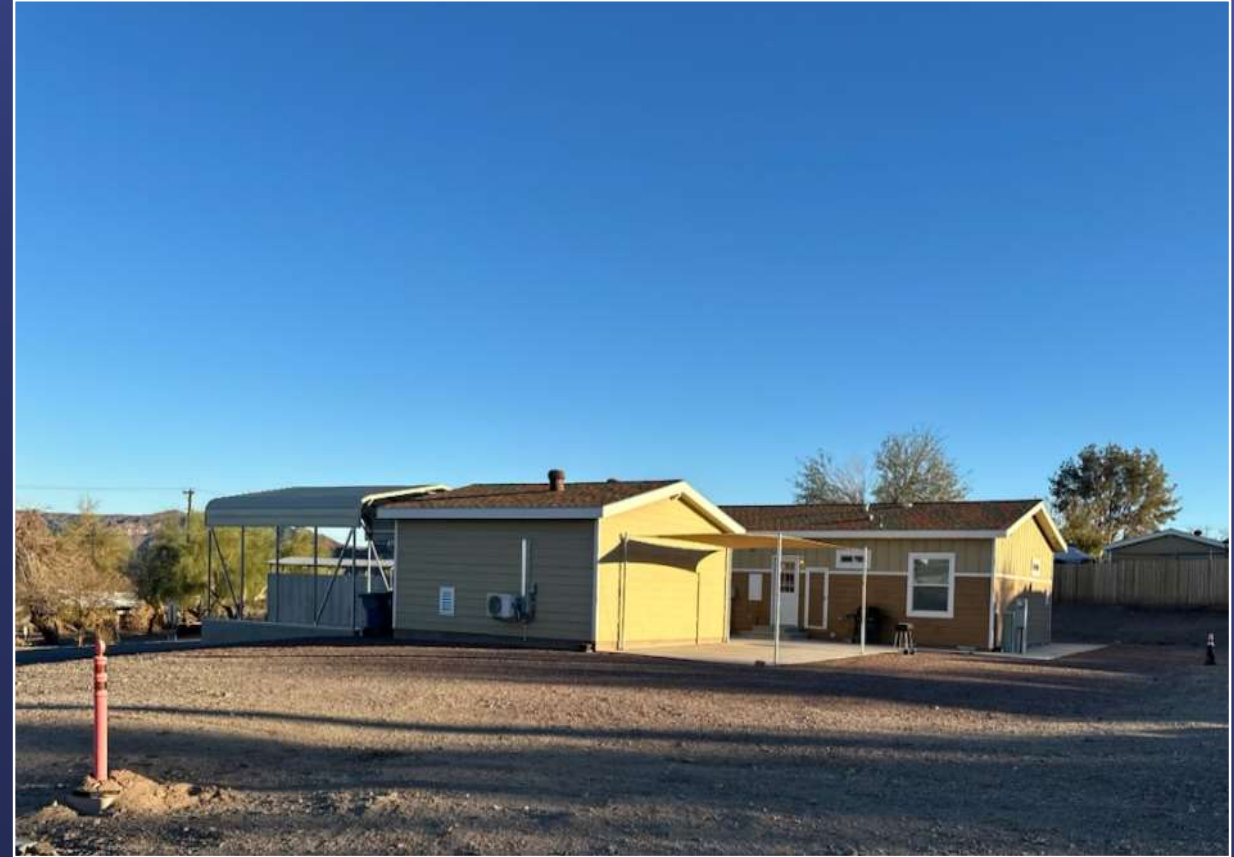
Perimeter Fencing w/Privacy Slats (68 houses)
