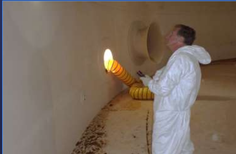
Tank Lining Inspection
