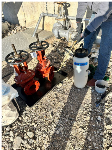
Staff disinfecting valves before installation on the potable water system
