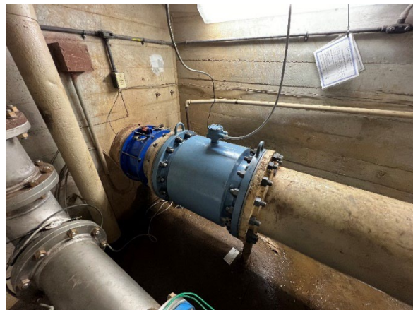
Staff removing and replacing a faulty meter with a new meter at WB-06 service connection on the Palos Verdes Feeder
