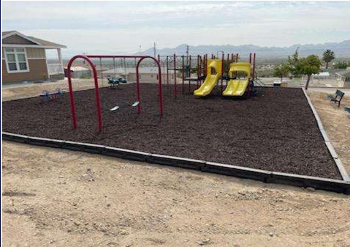
Playground Shade Structure and Fencing (Hinds Village, Eagle Mtn., Iron Mtn.)
