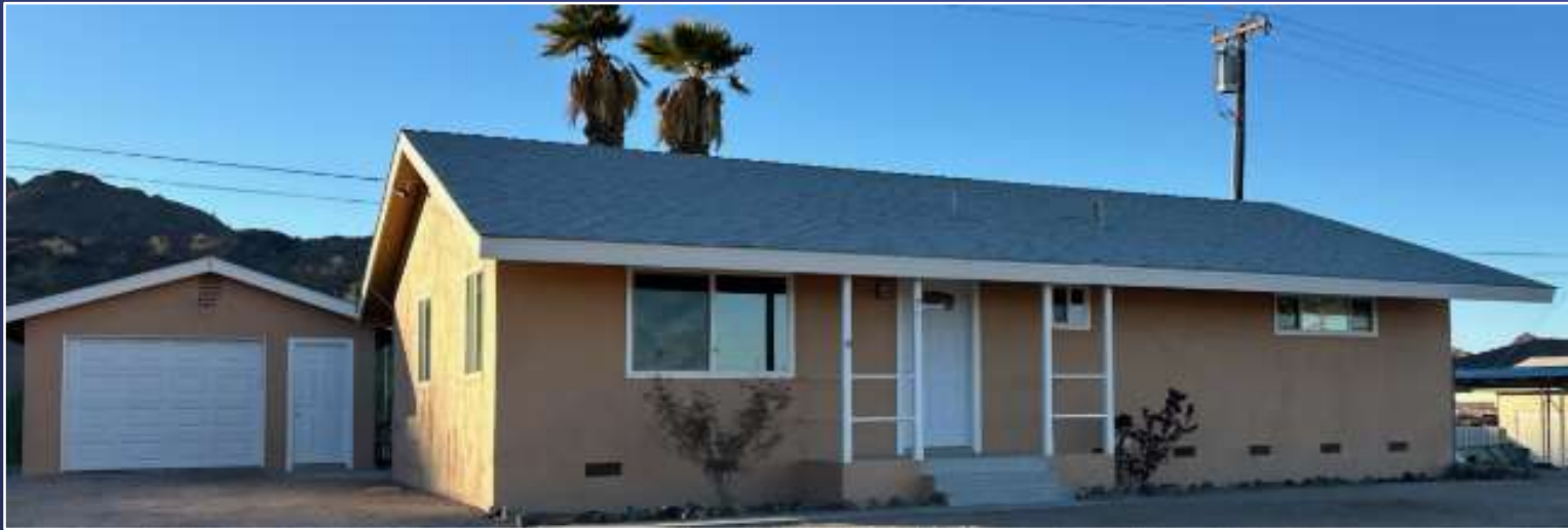
Exterior Paint and Windows
