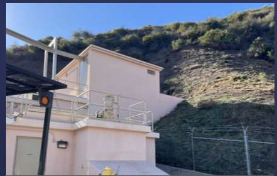
Cleared vegetation for defensible space
