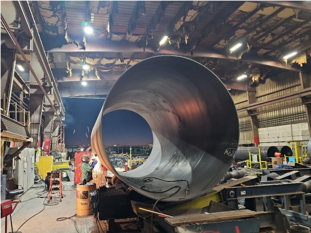
Lakeview Pipeline Procurement—Inspection of 117-inch Diameter Pipe Fabrication
