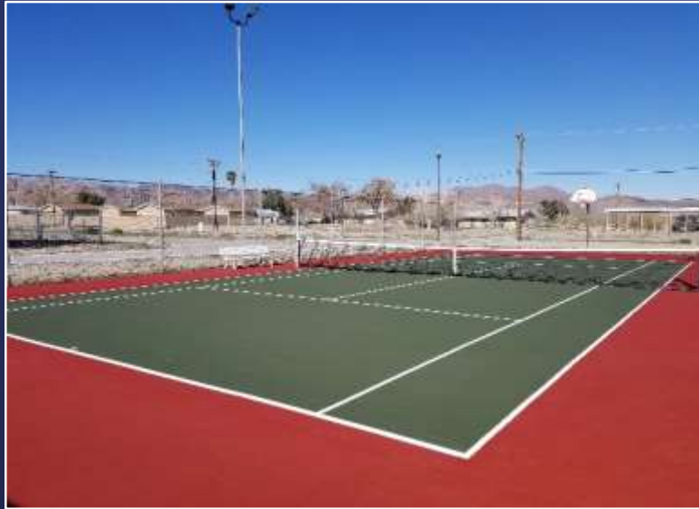
Resurfaced Sports Courts
