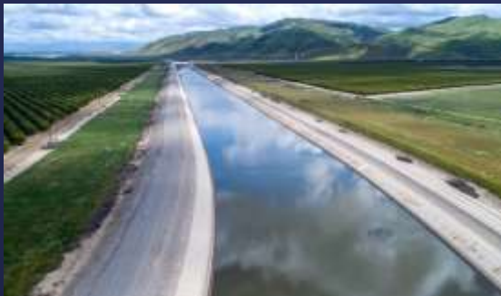
California Aqueduct in Central California
