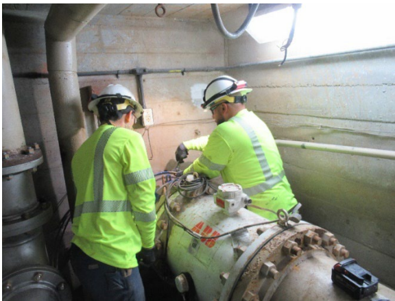
Staff removing and replacing a faulty meter with a new meter at WB-06 service connection on the Palos Verdes Feeder
