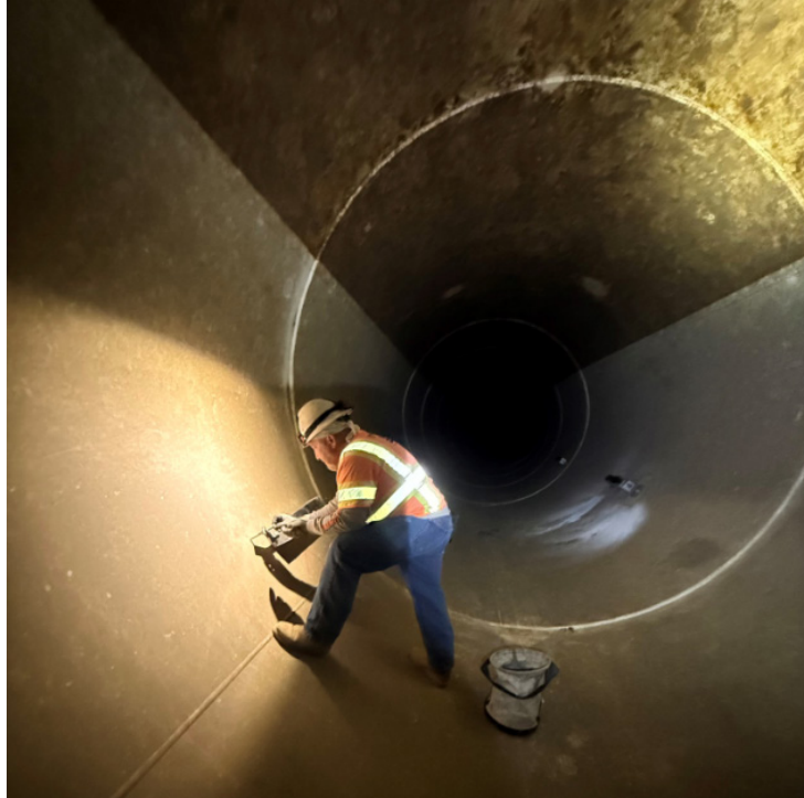
Wadsworth Bypass — Installing New Anode on the Eastside Pipeline
