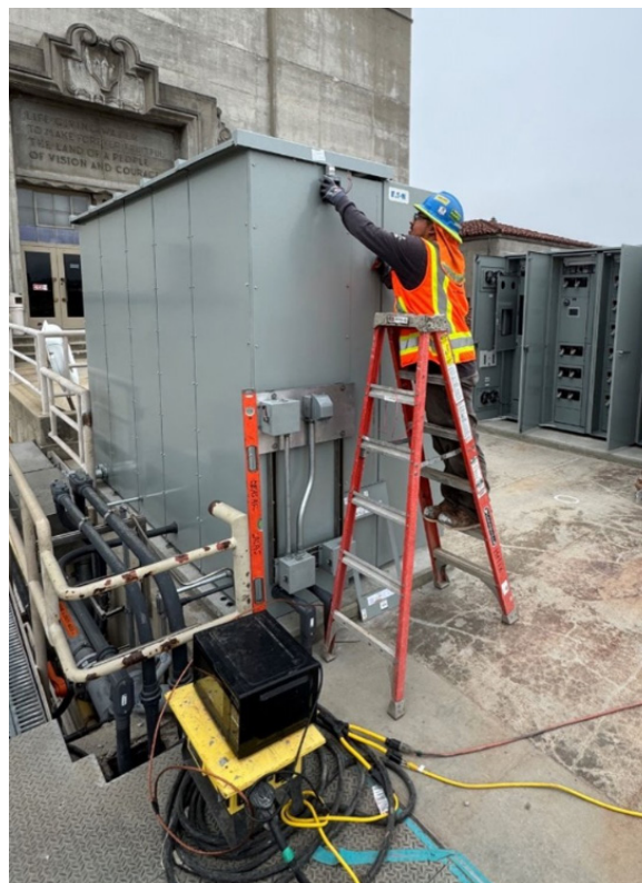
Weymouth Basins 5–8 and Filter Building No. 2 Rehabilitation Installing Lighting Photocell at New MCC, South of Basin 3
