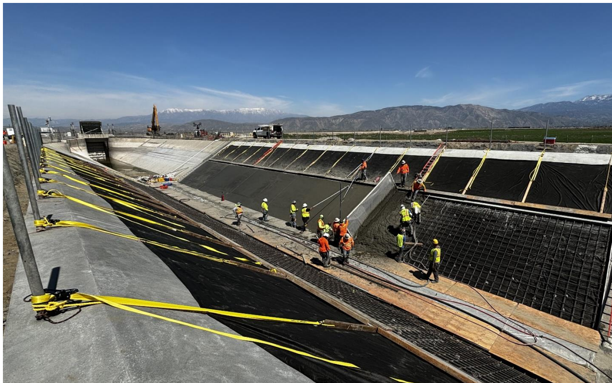
New canal panel concrete placement at Site 236 of San Diego Canal
