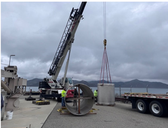
Assembly of DVL sleeve valve gate and inner sleeve
