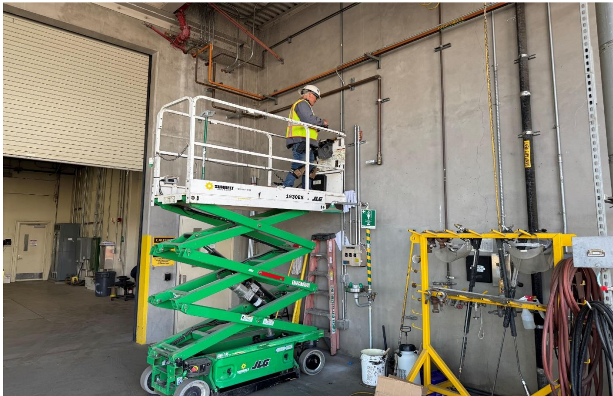
Installation of safety shower and eyewash in the coating shop at La Verne
