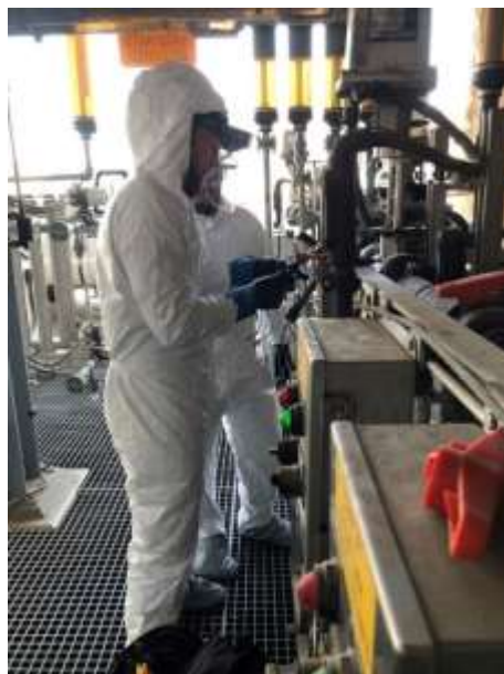
Staff performing electrical testing on a chemical flow meter at the Skinner plant
