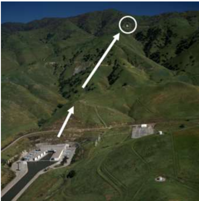
Figure 1—Annotated photo indicating the 1,926-ft lift that the 14 pump units at A. D. Edmonston Pumping Plant have to achieve.
