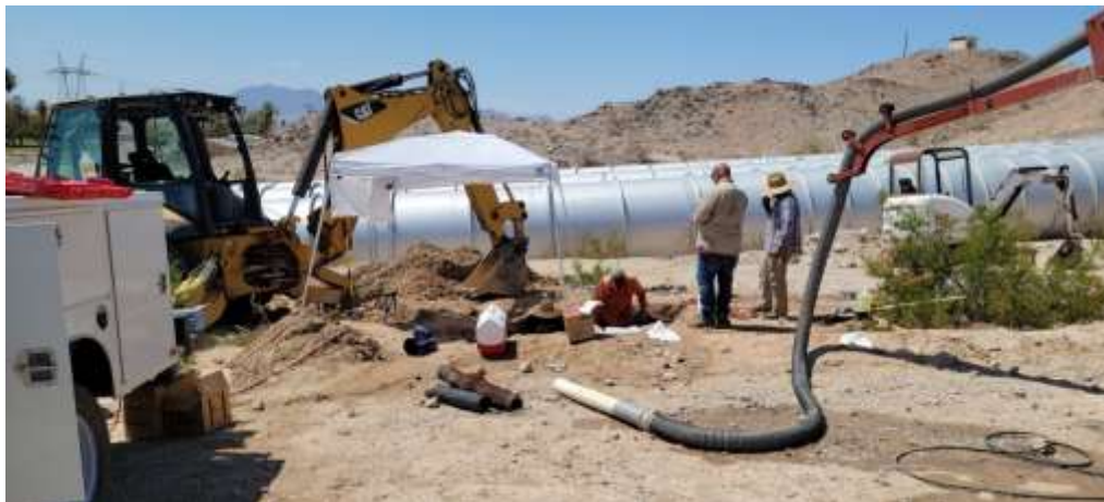
Staff repairing the domestic water line at Iron Mountain pumping plant
