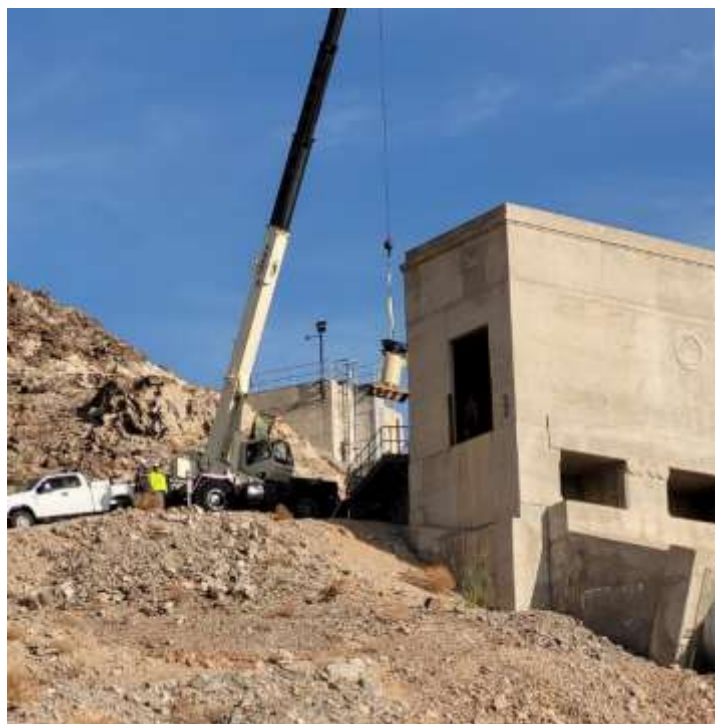
Staff replacing the air compressor at Iron Mountain pumping plant
