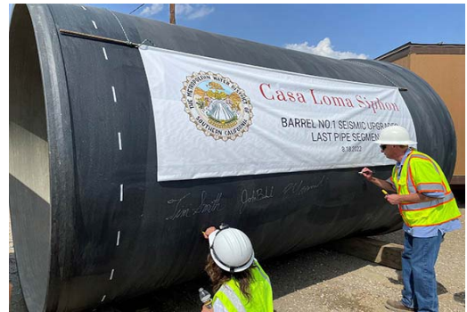
Casa Loma Siphon project to increase seismic resilience
