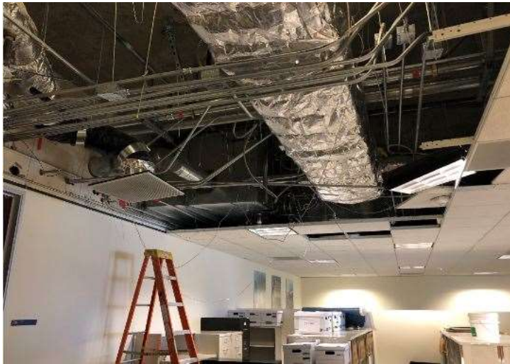
Headquarters Building Improvements—3 rd Floor Heat Pump Installation
