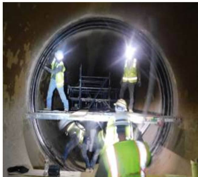
Freda Siphon Weko Seal Installation
