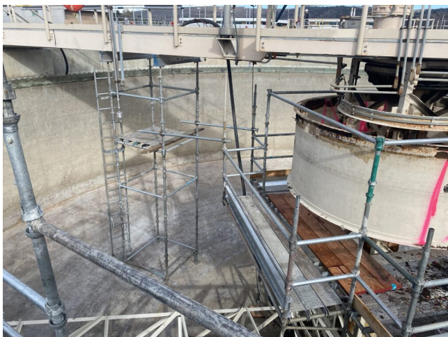
Scaffolding for work access (left) and staff performing weld repairs (right) at the Diemer solids thickeners
