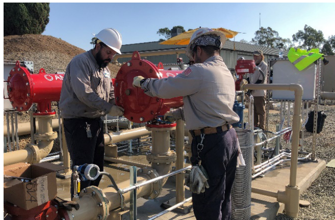
LACSD staff installing snail mitigation equipment at the Napolitano Innovation Center
