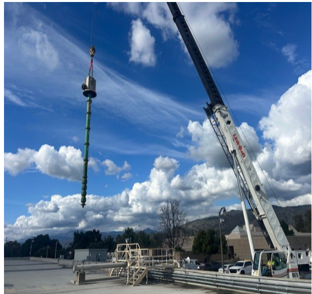
Staff performing spray disinfection (left) and installing a domestic water pump (right) at the Weymouth Finished Water Reservoir
