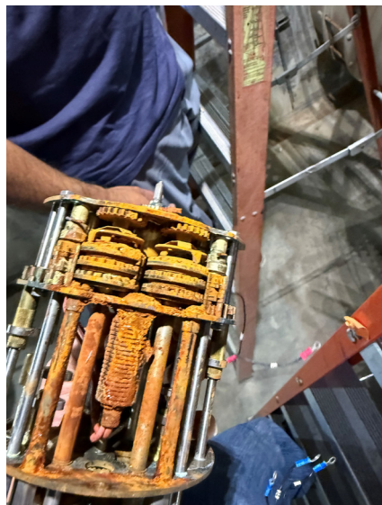
Filter valve actuator showing sediment buildup, requiring thorough cleaning and refurbishment
