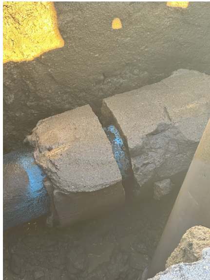
Staff coordinating with contractor to excavate a leaking water line at the Diemer facility
