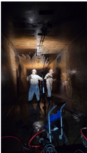
Staff pressure washing the filter effluent channel (left) and repairing ammonia injection equipment (right) at the Mills plant
