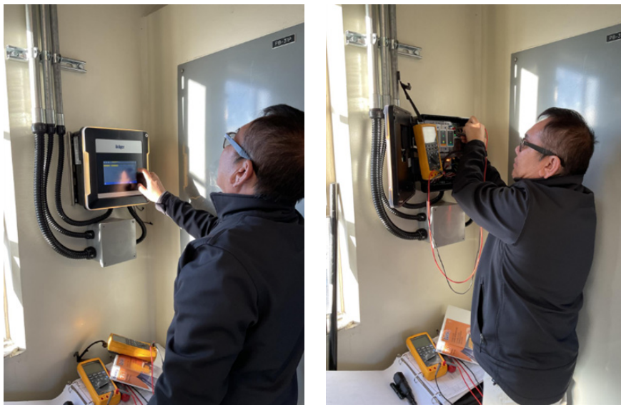
Staff programming chlorine leak detection panel and ensuring all connections and voltages are correct
