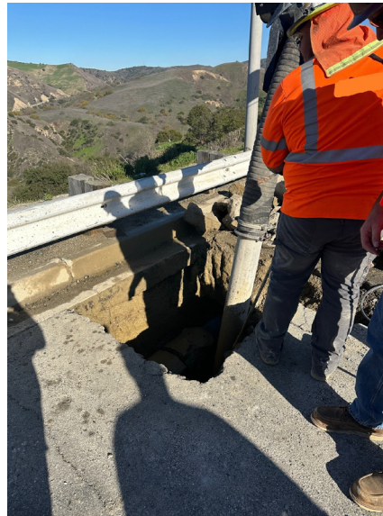
Staff coordinating with contractor to excavate a leaking water line at the Diemer facility
