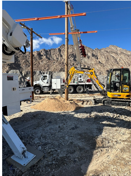
Staff replacing power poles at the Iron Mountain pump plant
