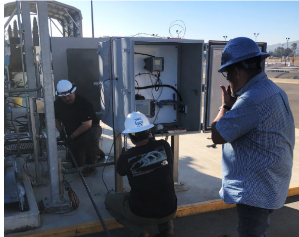
Staff building sampling skids for pathogen testing at the Napolitano Innovation Center
