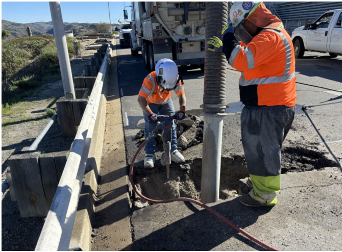
Vendor assisting staff with vac truck services (left) and staff locating water line (right) at Diemer facility
