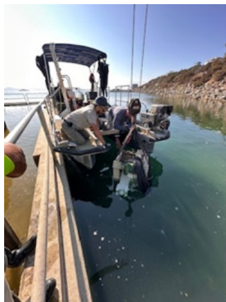
Refurbished actuator (left) and installation of refurbished actuator at Lake Mathews outlet tower (middle and right)
