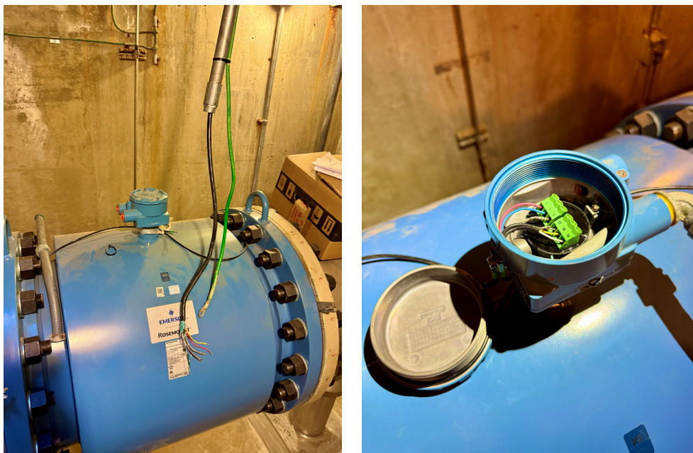
Service connection magnetic flow meter spool (left) and wiring connection (right)
