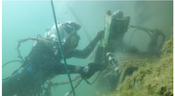
As-found condition of existing Tier 1 actuator (left) and actuator pressure washing (right)
