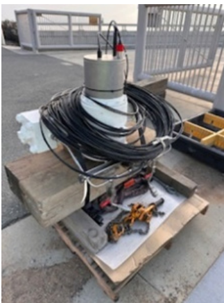
Refurbished actuator (left) and installation of refurbished actuator at Lake Mathews outlet tower (middle and right)
