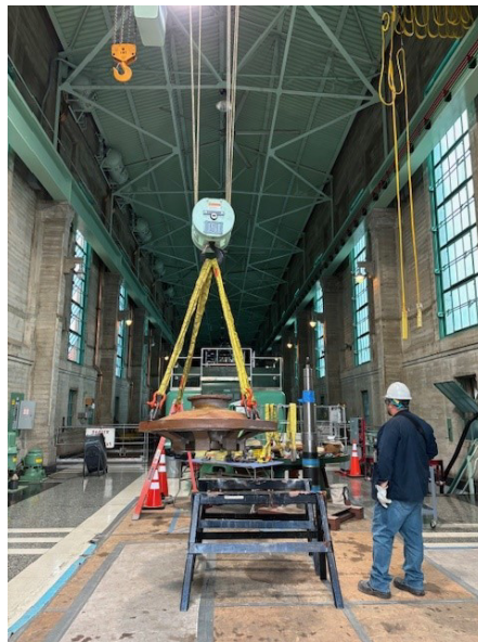
Staff working on Gene Unit 1 discharge valve
