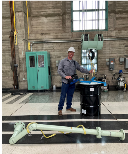
Staff removing and replacing a section of cooling water pipe at the Intake pump plant
