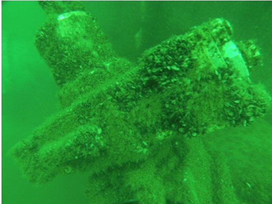
As-found condition of existing Tier 1 actuator (left) and actuator pressure washing (right)
