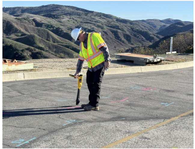
Vendor assisting staff with vac truck services (left) and staff locating water line (right) at Diemer facility
