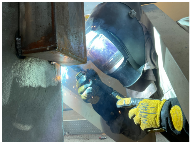
Scaffolding for work access (left) and staff performing weld repairs (right) at the Diemer solids thickeners
