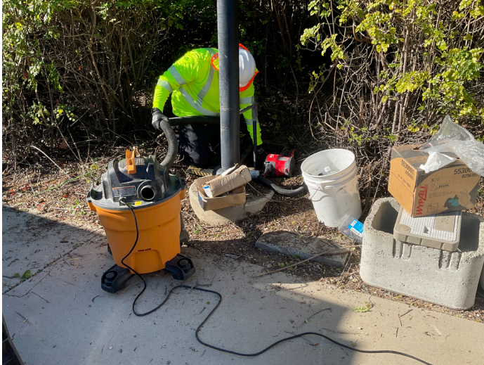
Clearing the electrical conduit (left) and preparing new wire for installation (right)
