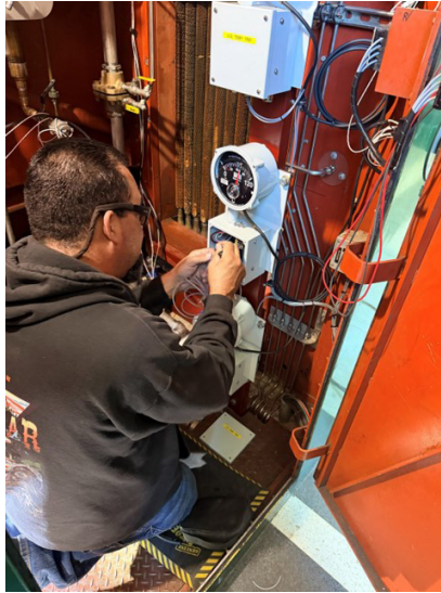
Staff calibrating new bearing temperature devices at Eagle Mountain pump plant
