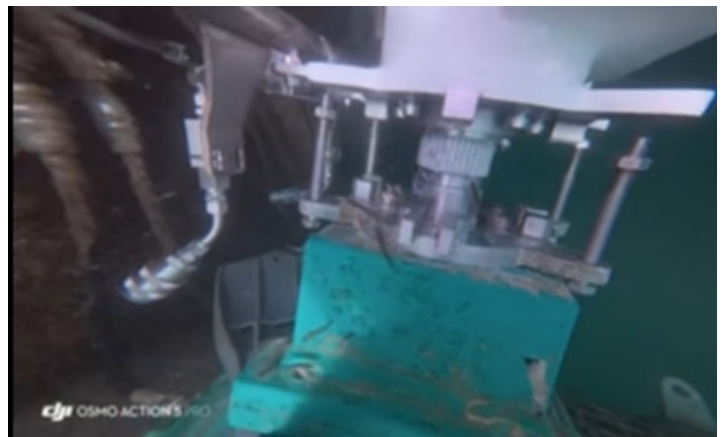
Refurbished actuator (left) and installation of refurbished actuator at Lake Mathews outlet tower (middle and right)
