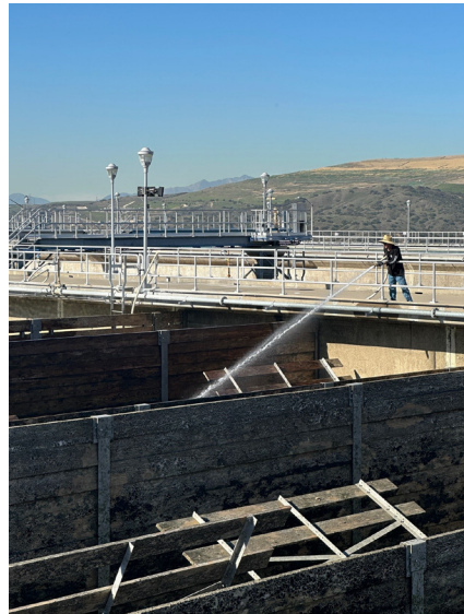
Staff washing down a sedimentation basin at the Diemer plant
