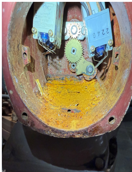
Filter valve actuator showing sediment buildup, requiring thorough cleaning and refurbishment
