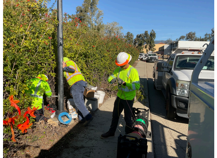
Clearing the electrical conduit (left) and preparing new wire for installation (right)
