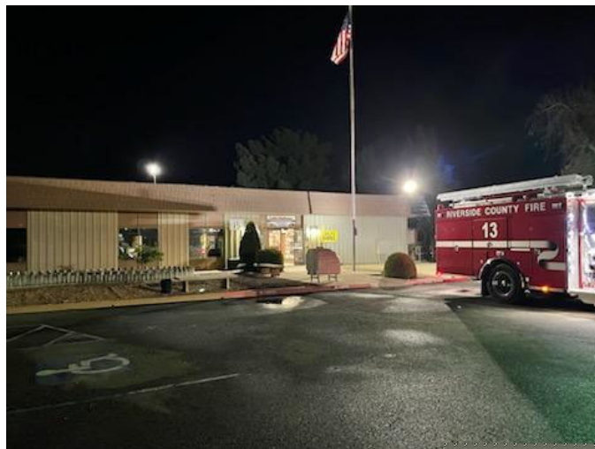
Tin Fire at Lake Mathews Administration Building
