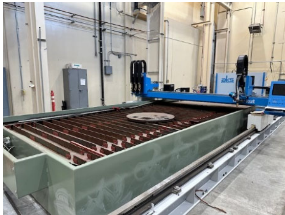
New Plasma Arc Cutting System Installation In-Progress
