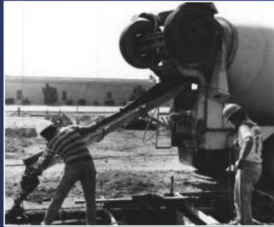
Pouring concrete for Water Quality Lab, 1983
