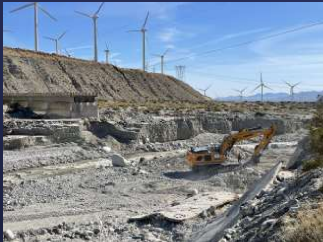
Whitewater Bridge Demolished
